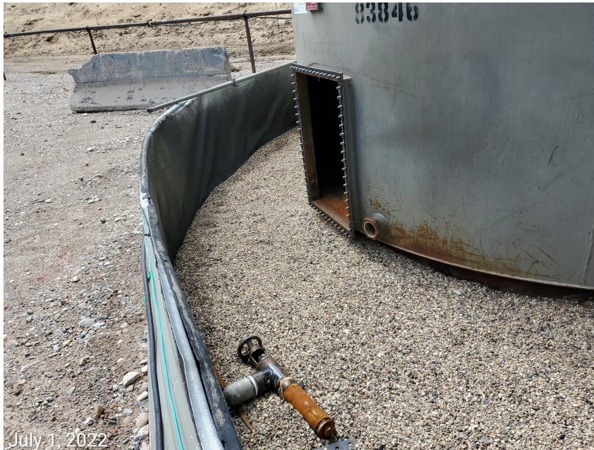
Photo 2: Photo taken from the northeastern-most tank. Stained soils appear to have been cleaned and Work at tank appears to be in process, however it is unclear if corrective actions have been addressed in its entirety; manway cover removed, pipes leading to tank have been disconnected; liner integrity beneath tank unknown.
