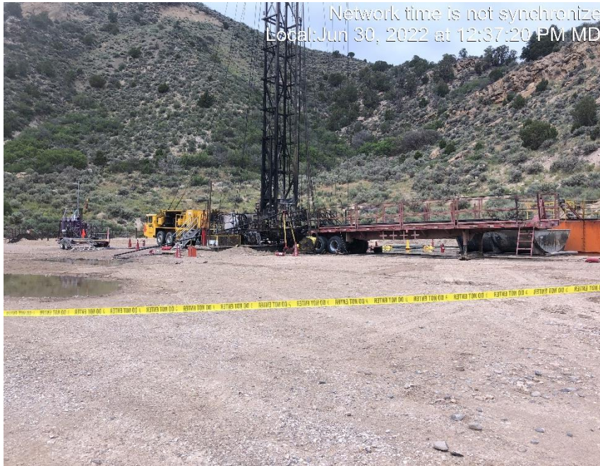
Photo #7053 Work over rig fire.
