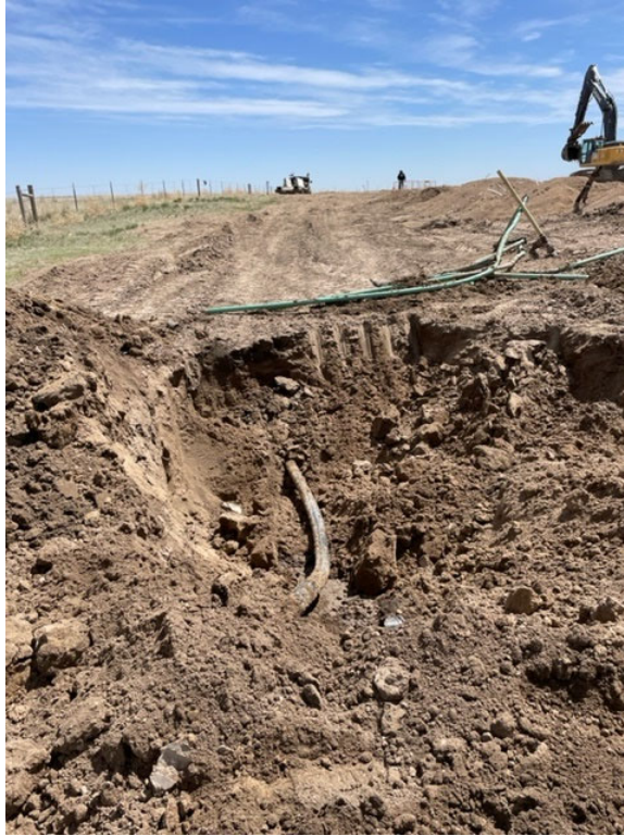
9 – Kummer PC LE 23-99HZ flow and dump lines in a common trench approaching the east side of the former tank pad
