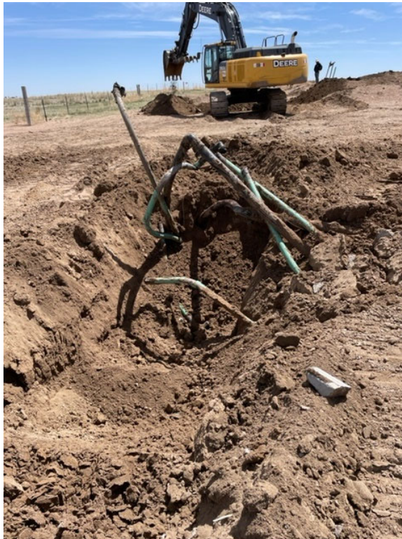
8 – Kummer PC LE 23-99HZ flow and dump lines in a common trench at the heater treater
