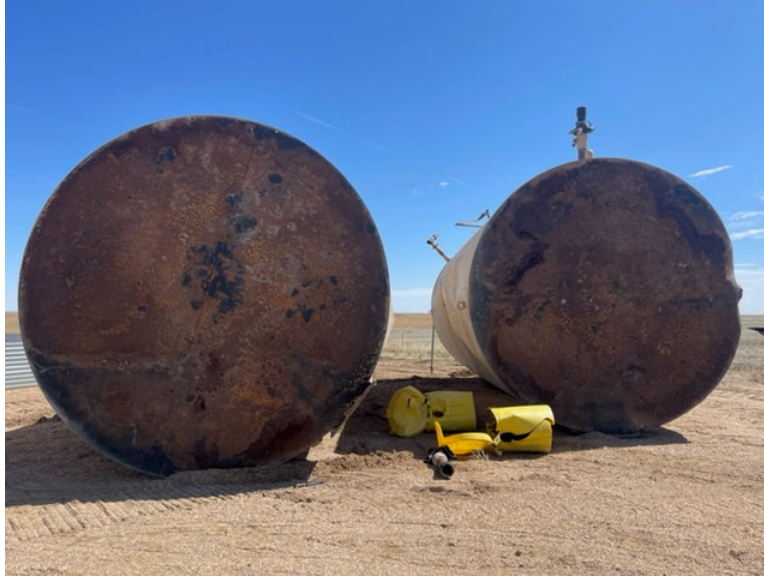
1 – Kummer PC LE 23-99HZ AST bases, rusted, no penetration
