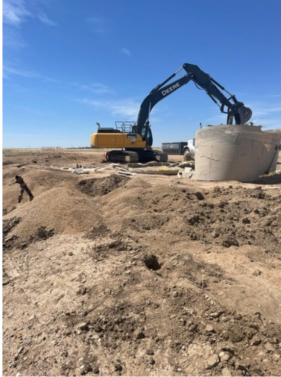
5 – Kummer PC LE 23-99HZ south above ground PWV crushed and removed during abandonment activities
