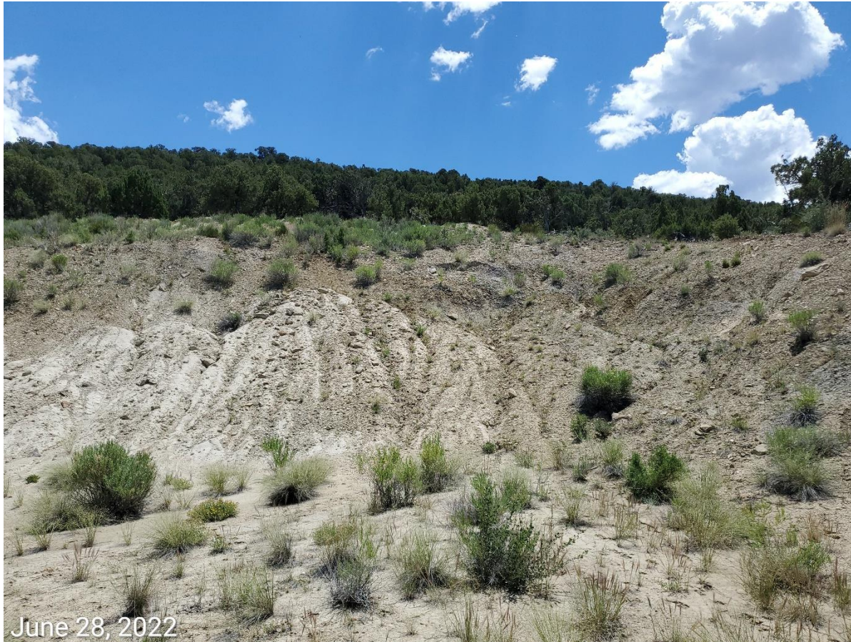
Photo 3: Photo taken from the cut slopes of the Location. Photo shows erosion degradation occurring on the slopes; BMPs to control stormwater in a manner that minimizes erosion and degradation are missing or insufficient on the Location
