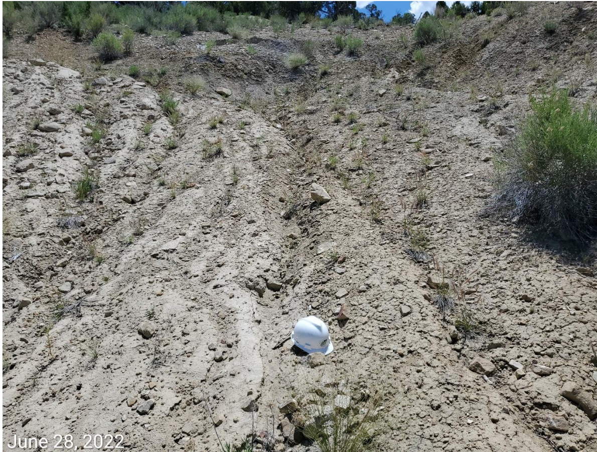
Photo 4: Continued from photo 3. . Photo shows erosion degradation occurring on the slopes . Hard hat for reference.
