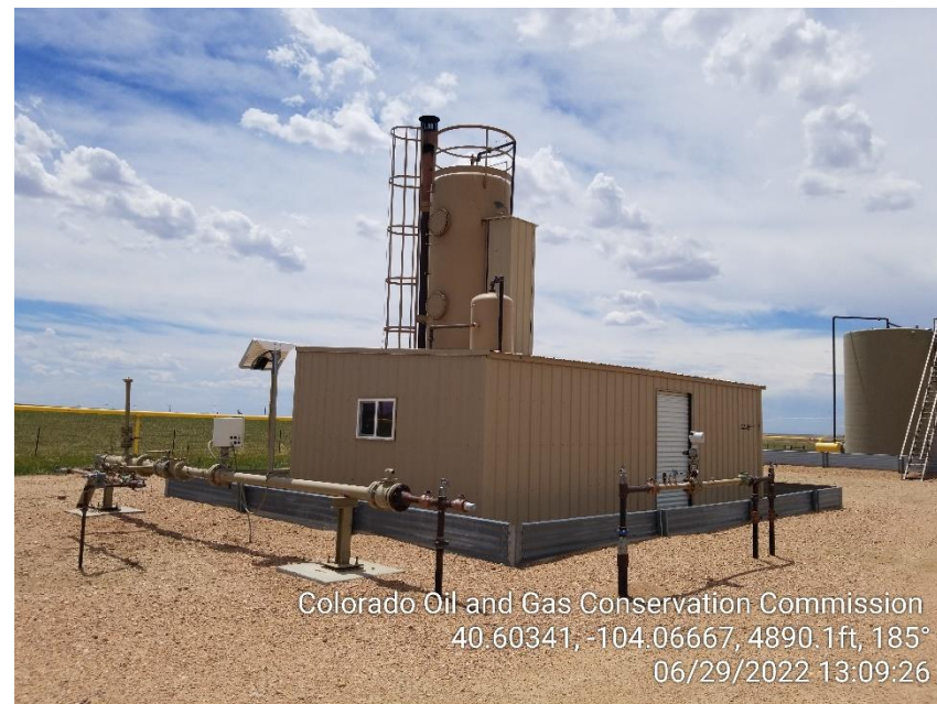
Photo 10 – Heater Treater and Gas Meters
