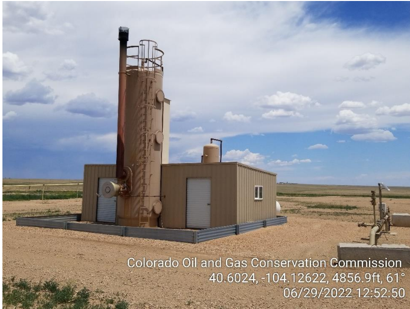
Photo 1 – Heater Treater and Gas Meters
