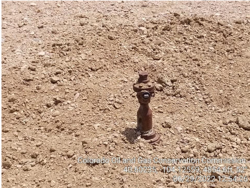
Photo 3 – Unmarked Riser at Wellhead
