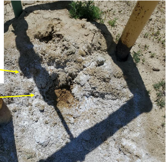
Photo 1: Photo shows riser observed on the west end of the Location, near the entrance. Fluids observed leaking from the riser resulting in a spill and impacts. Salt accumulation evident at point of release- middle photo taken from the 4/22/2021 inspection, and shows that the same accumulations are evident within past inspections, suggesting spill may have been on-going for at least a year
