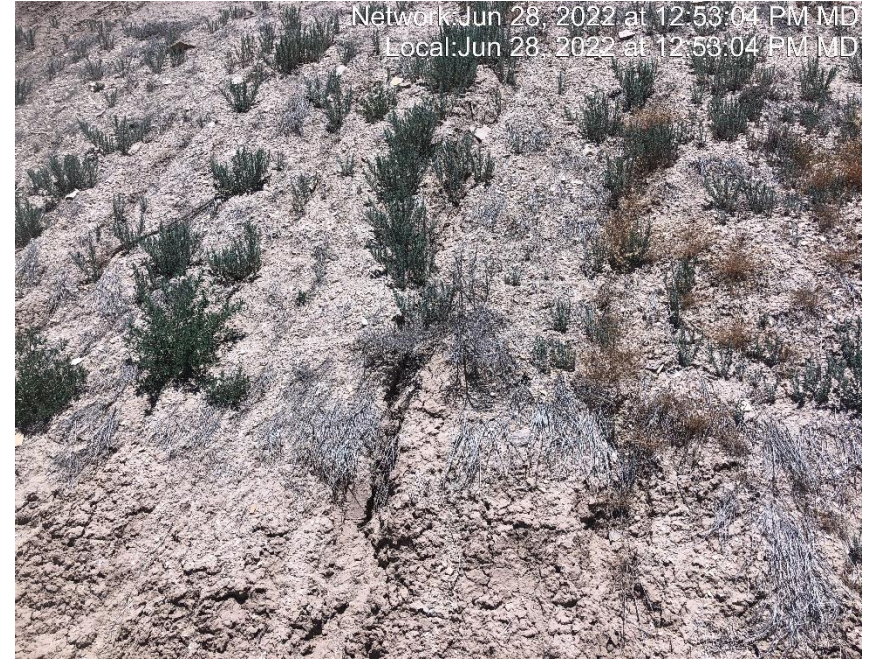
Photo #7002 Rill erosion occurring on cut slope.
