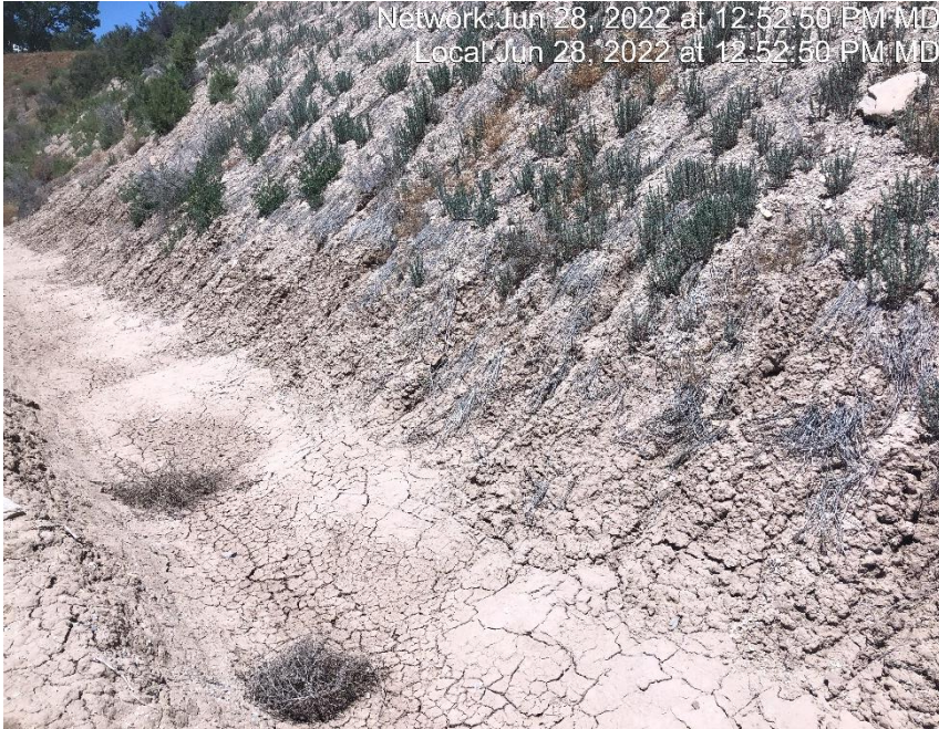
Photo #7001 Rill erosion occurring on cut slope.
