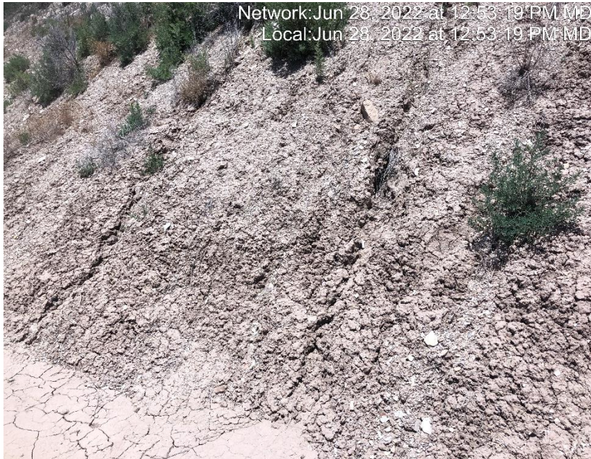
Photo #7003 Rill erosion occurring on cut slope.
