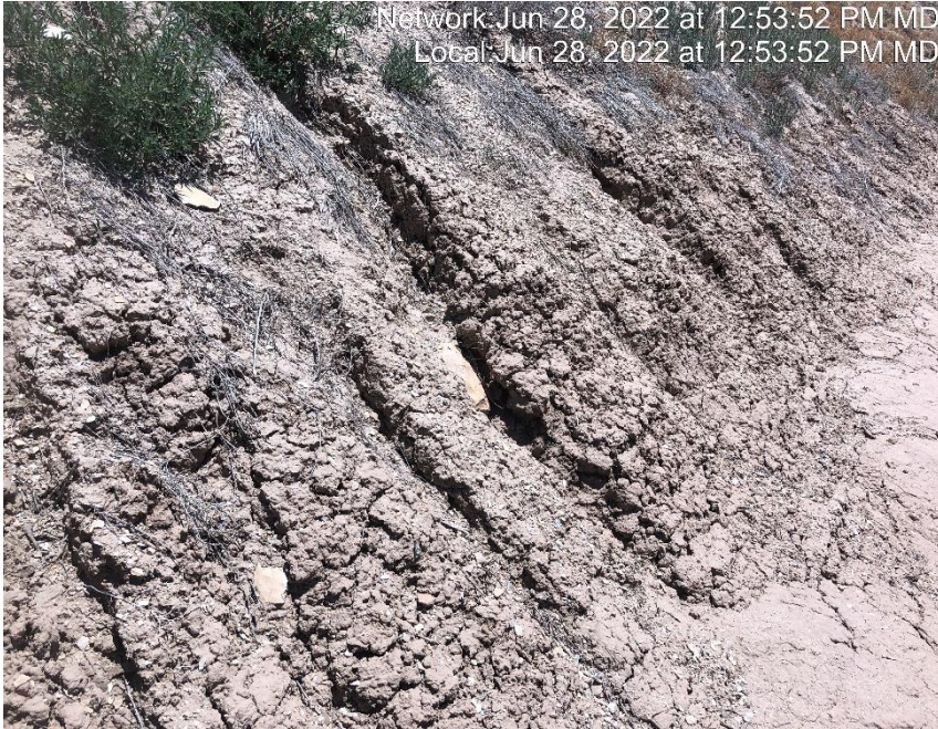
Photo #7006 Rill erosion occurring on cut slope.
