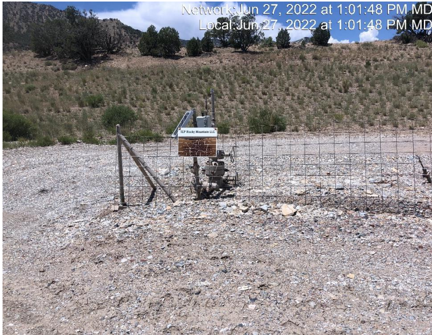
Photo #6977 Wellhead sign weathered and not legible.
