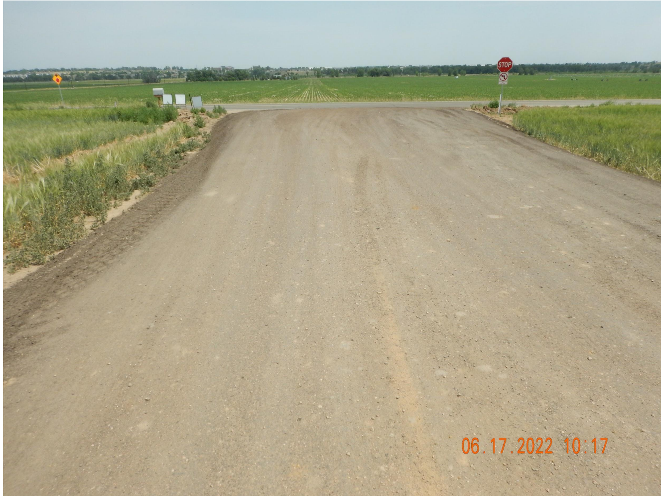
Photo 2. Photo taken from the entrance of location, facing North. Photo illustrates Operator added recycled asphalt as additional BMP.
