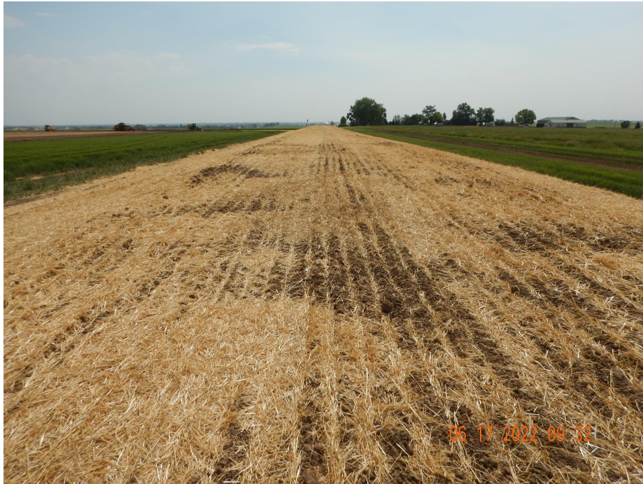
Photo 4. Photo taken from the western topsoil stockpile, facing East. Operator has seeded and straw crimped mulch into the topsoil.
