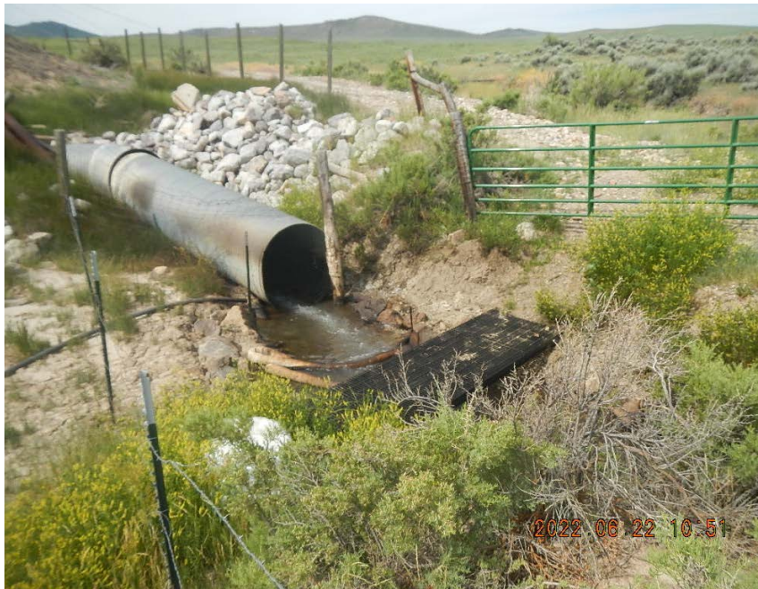
Boom at Pit Facility ID: 116587 discharge. Oily stained vegetation observed and hydrocarbon odor noted.
