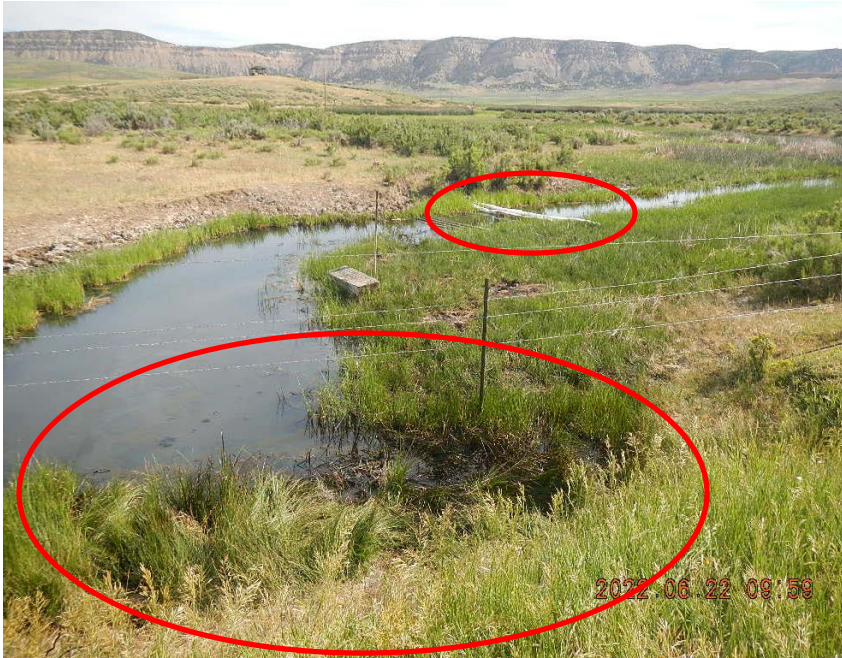
Outfall of culvert beneath County Road LY5. Oily impacted vegetation and oil observed on the water surface. Booms are placed down gradient.
