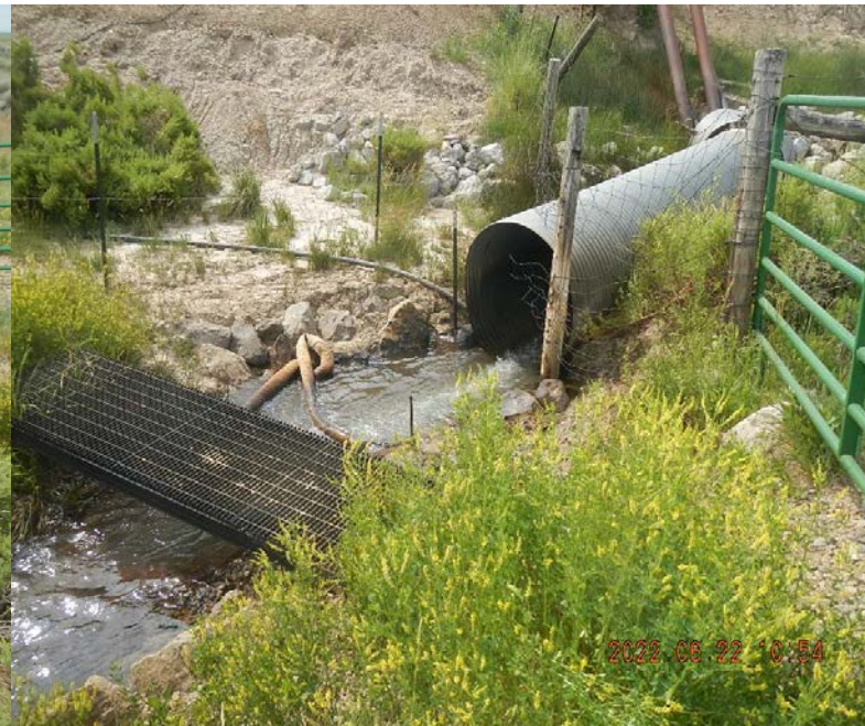
Boom at Pit Facility ID: 116587 discharge. Oily stained vegetation observed and hydrocarbon odor noted.
