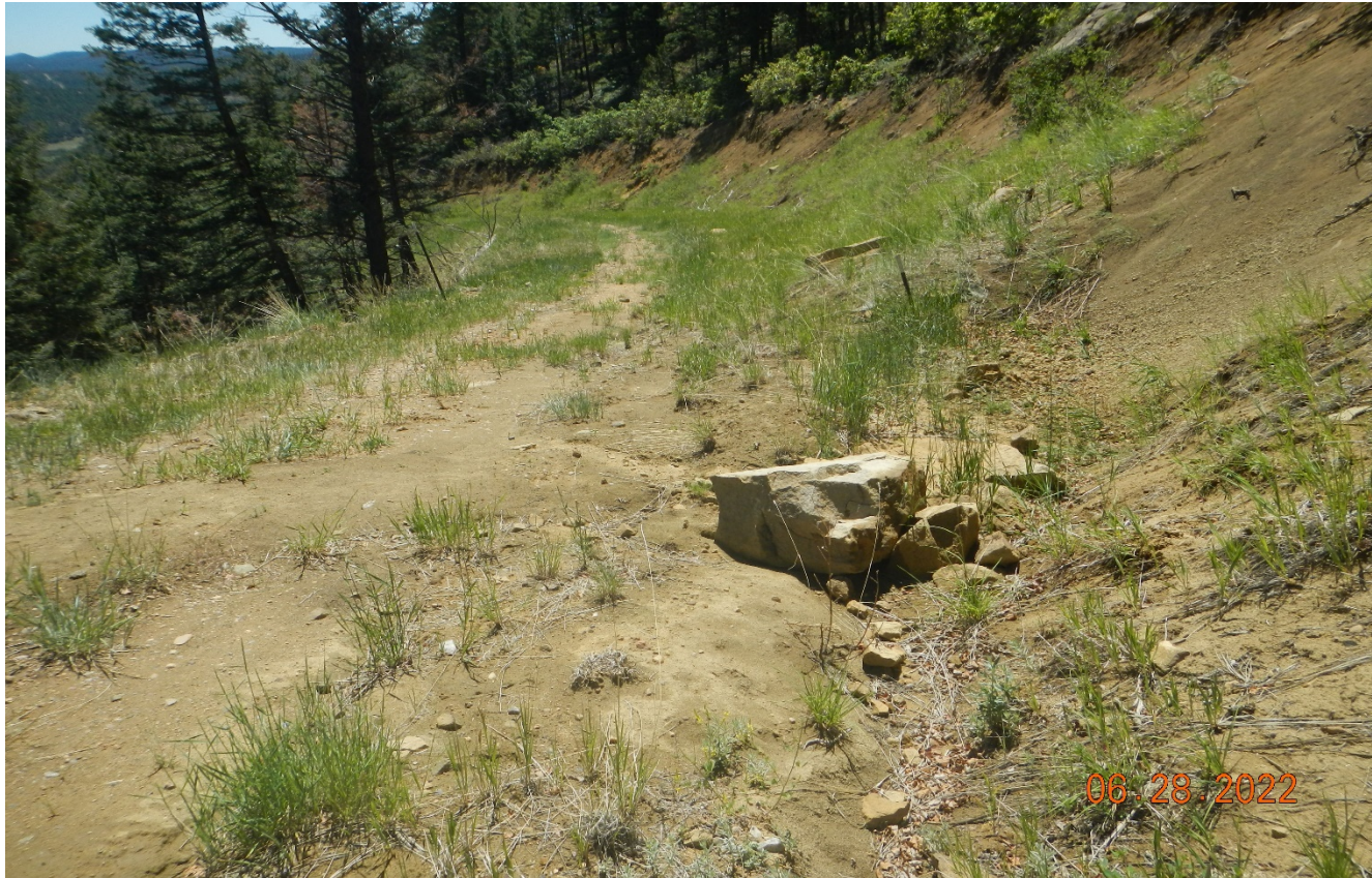
Photo 2. Facing east along the access road. There are a few culverts that are filled in with sediment and stormwater is not properly diverted that need maintenance. (Perhaps handwork can be performed to prevent disturbance.)
