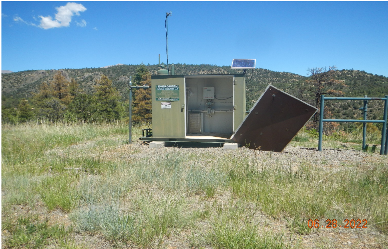
Photo 4. The door is hanging off and needs to be repaired.
