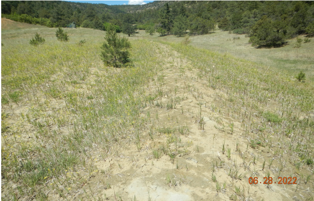
Photo 6. Facing west along the fill slope of the location which will need to be recontoured back into the cut slope.
