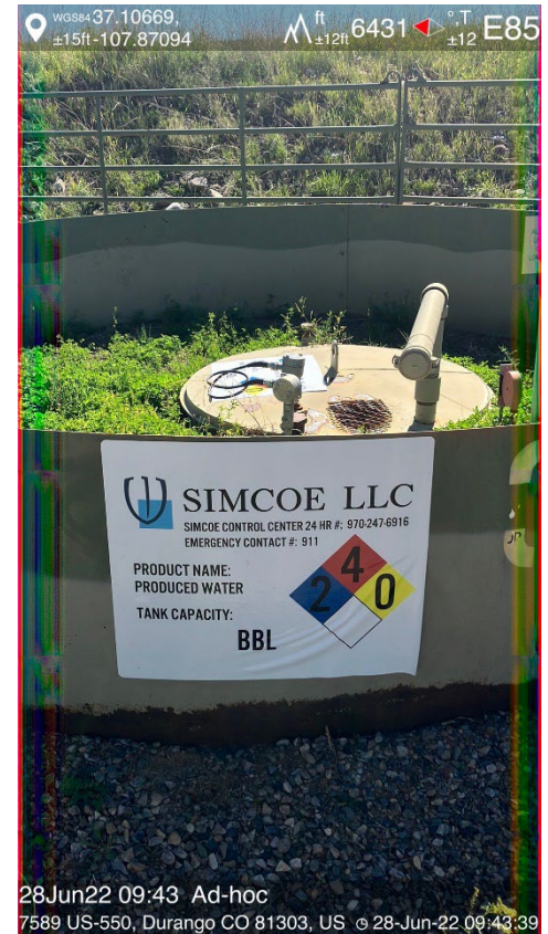
IMG 02 Tank label with no capacity
