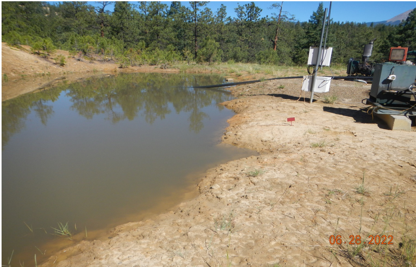
Photo 2. The water level is at 2 ft. freeboard and needs to be lowered.
