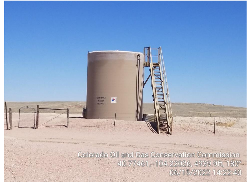
Photo 2 – Produced Water Tank
