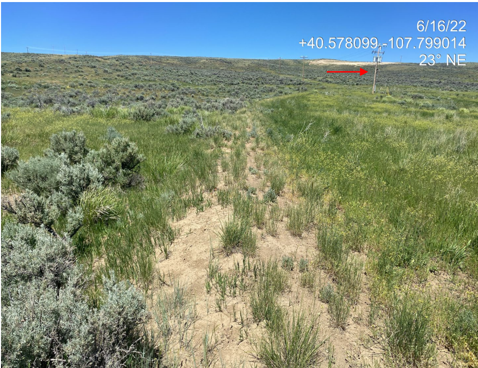
Photo 6. Photo taken from the west of the Location shows the Location has not been recontoured; the Location perimeter berm remains. Note also the power line (red arrow) associated with the Location which must be removed per Rule 1004.a.
