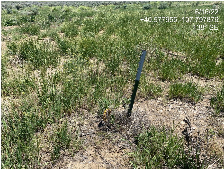
Photo 14. Photo taken from the southeast of the Location shows a guy line anchor which must be removed per Rule 1004.a.
