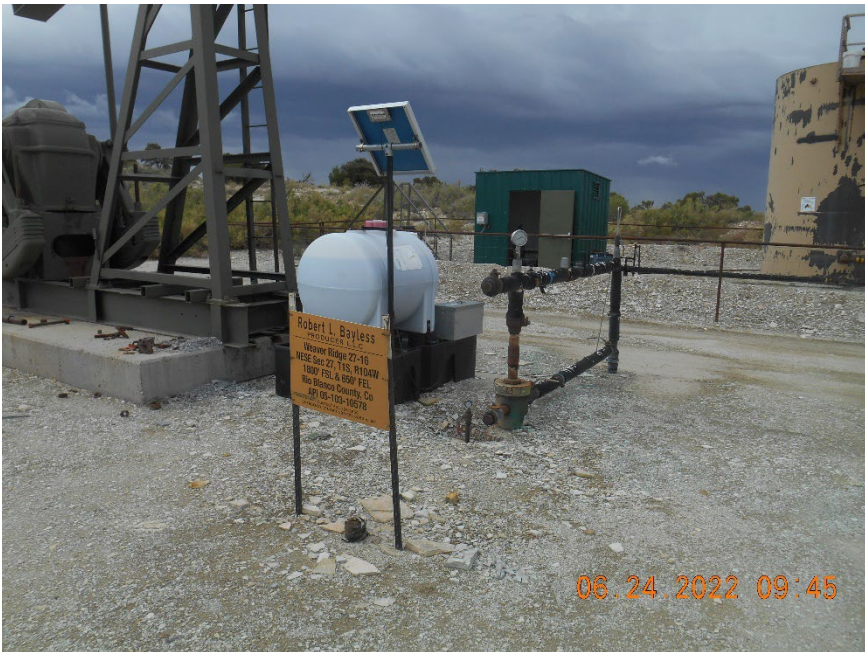
Injection wellhead with sign.
