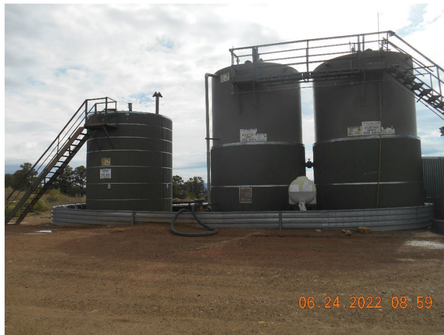
Tank battery and Secondary containment of chemicals
