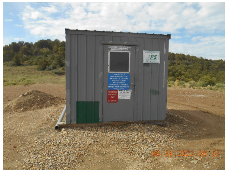
Injection wellhead housing with sign
