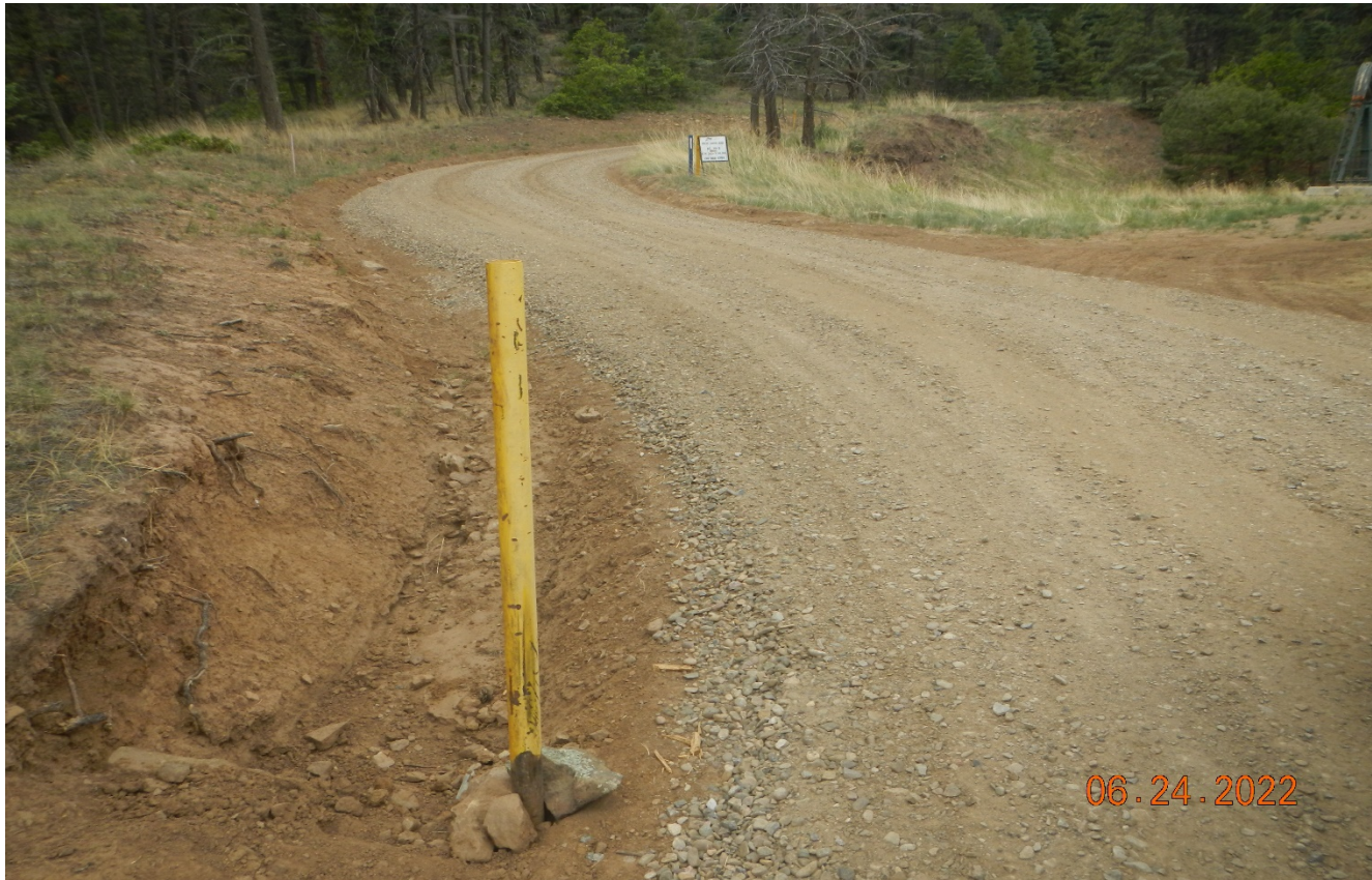
Photo 2. Facing along the access road near the location. There has been additional gravel spread along the road and the culverts are maintained.
