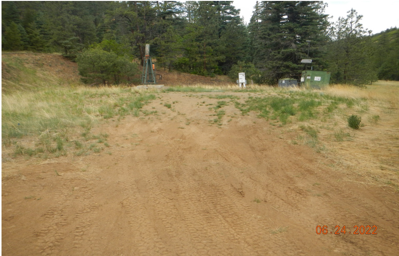
Photo 3. Facing toward the well site.
