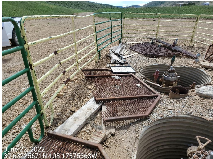
Photo 6: Photos taken from the TA wells on the east end of the Location. Photo shows uncovered cellars/pipes, and well signs in disarray. Photo also shows wood and trash debris
