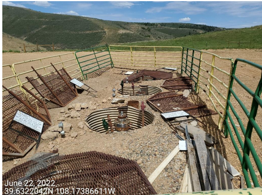
Photo 5: Photos taken from the TA wells on the east end of the Location. Photo shows uncovered cellars/pipes, and well signs in disarray. Photo also shows wood and trash debris
