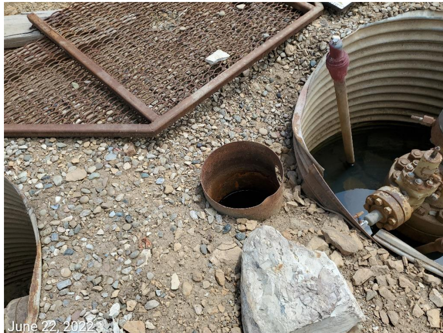
Photo 6: Photos taken from the TA wells on the east end of the Location. Photo shows uncovered cellars/pipes, and well signs in disarray. Photo also shows wood and trash debris
