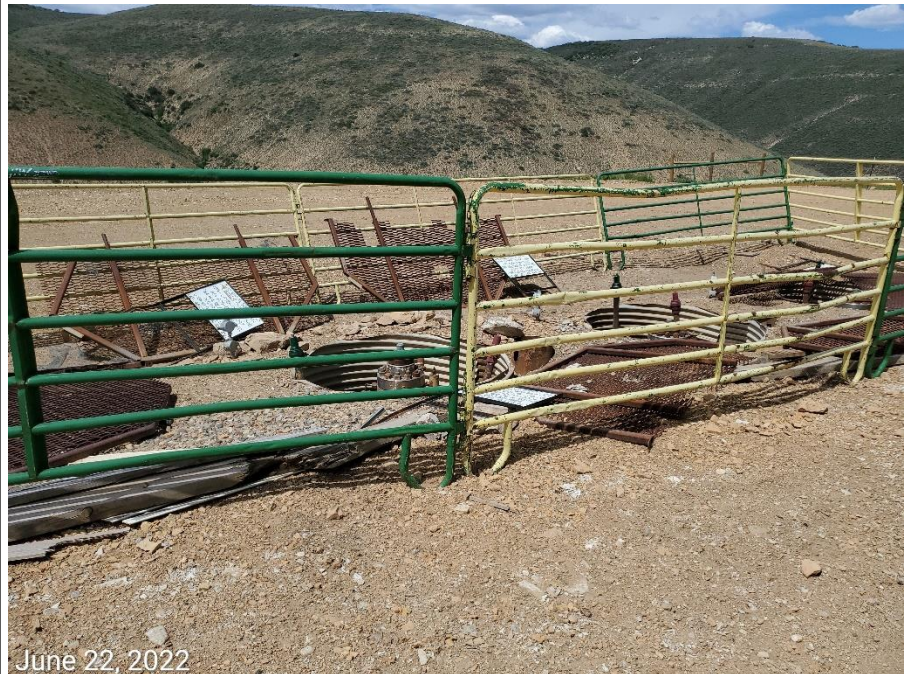
Photo 5: Photos taken from the TA wells on the east end of the Location. Photo shows uncovered cellars/pipes, and well signs in disarray. Photo also shows wood and trash debris
