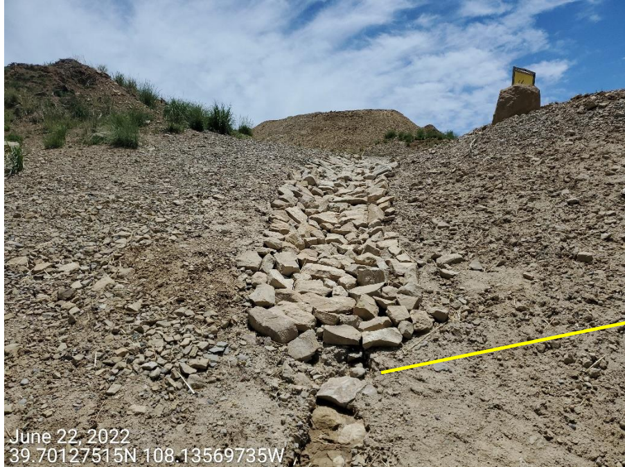
Photo 1: Photos taken from the sediment trap on the north end of the Location. Photo shows additional work to the inlet has been performed, however, inlet does not appear to have been constructed with geotextile lining per good engineering practices, and degradation to the control is recurring (arrow).
