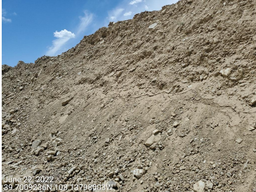
Photo 4: Photos example showing BMPs to minimize erosion and degradation on slopes of the Location remain missing or insufficient.
