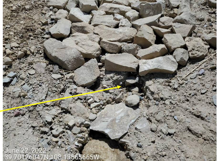
Photo 1: Photos taken from the sediment trap on the north end of the Location. Photo shows additional work to the inlet has been performed, however, inlet does not appear to have been constructed with geotextile lining per good engineering practices, and degradation to the control is recurring (arrow).
