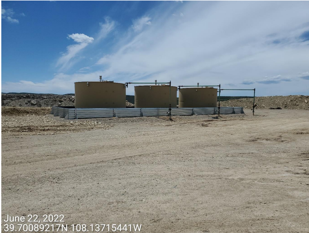
Photo 10: Signage and labels missing from battery, and tanks.
