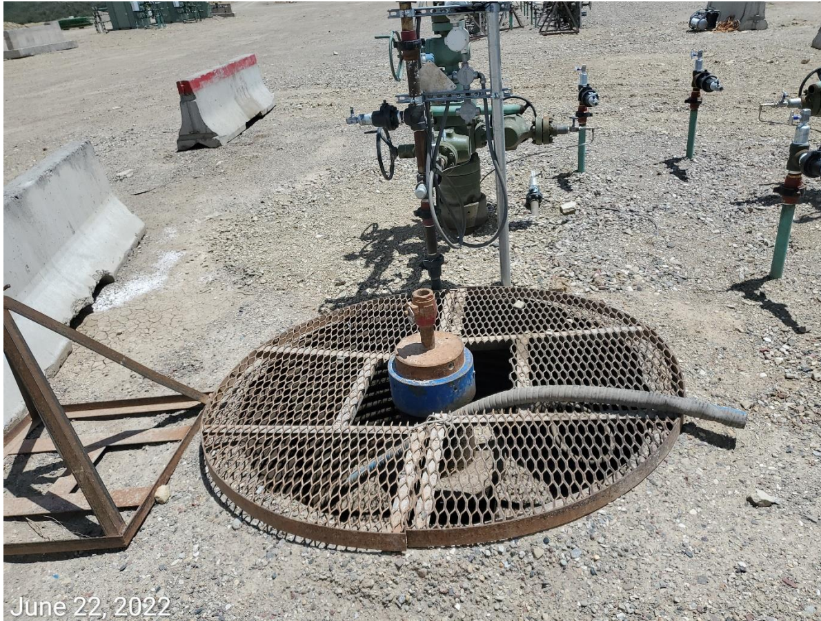
Photo 1: Photo shows equipment/cellar/conductor/etc.. remaining at the PA well site.
