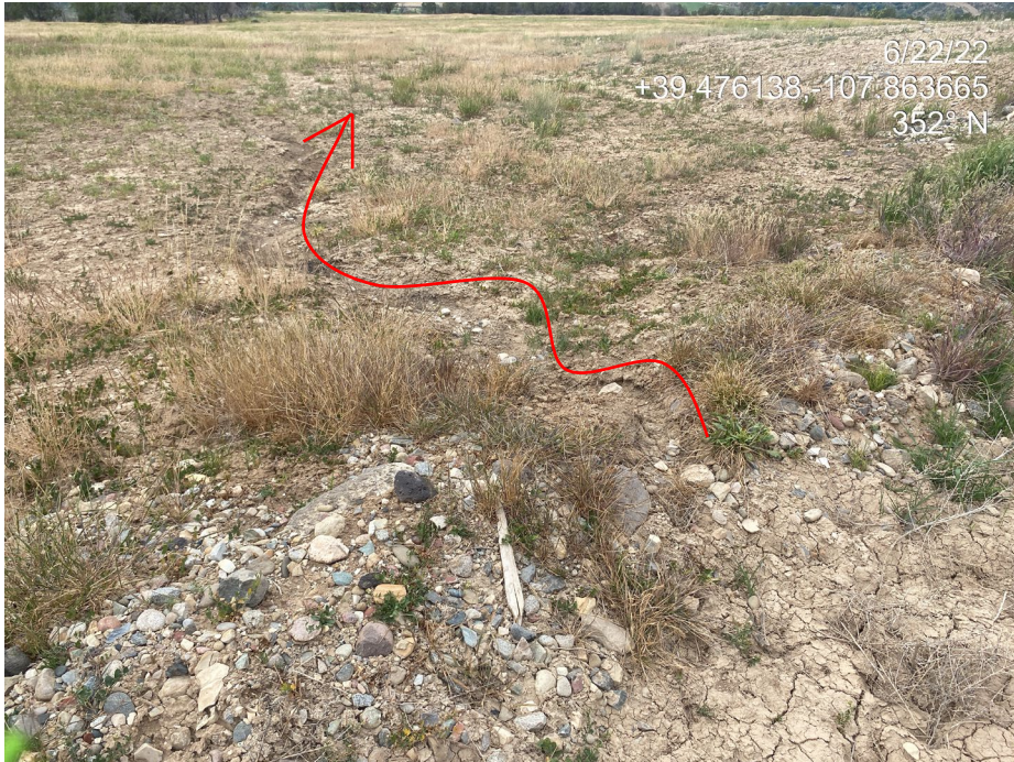
Photo 10. Photo taken from the west of the Location shows where stormwater has broken through a stormwater diversion ditch and is degrading adjacent interim areas.
