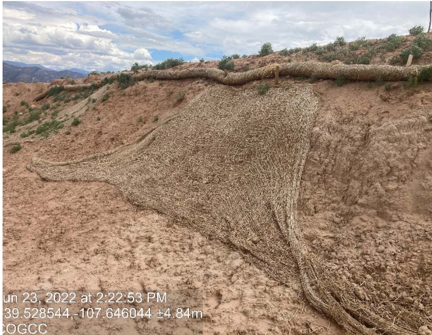
Lack of stabilization/ erosion/ debris
