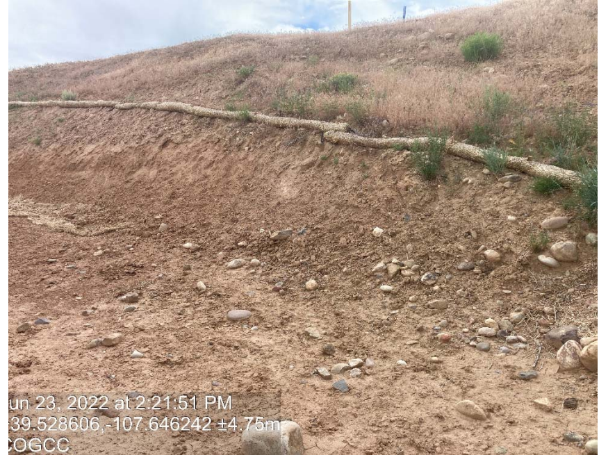
Lack of stabilization/ erosion
