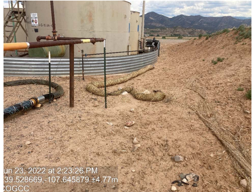
Lack of stabilization/ erosion/ debris
