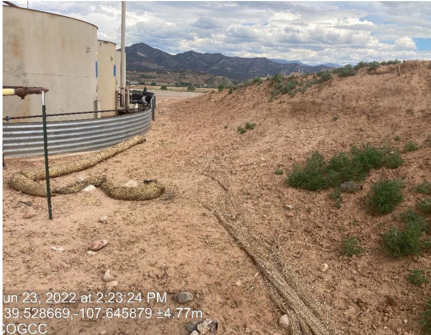
Lack of stabilization/ erosion/ debris
