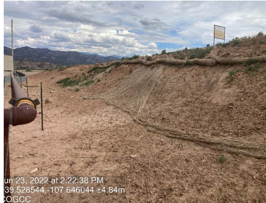
Lack of stabilization/ erosion/ debris
