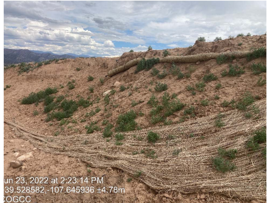
Lack of stabilization/ erosion/ debris
