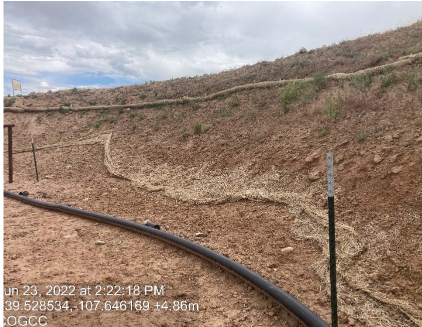
Lack of stabilization/ erosion/ debris
