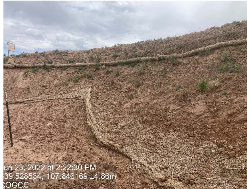
Lack of stabilization/ erosion/ debris
