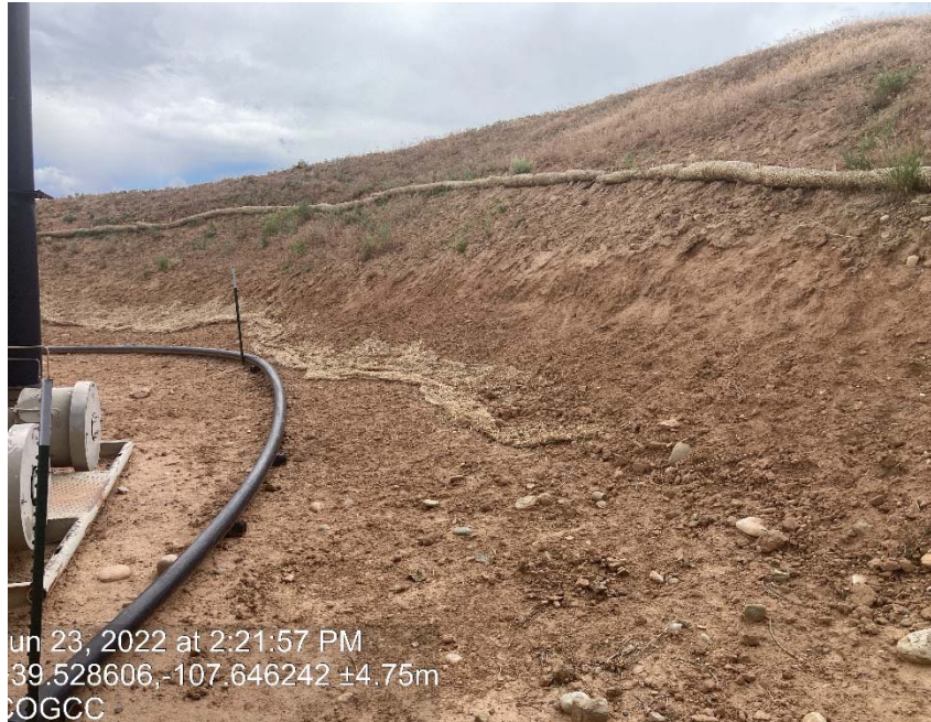
Lack of stabilization/ erosion/ debris
