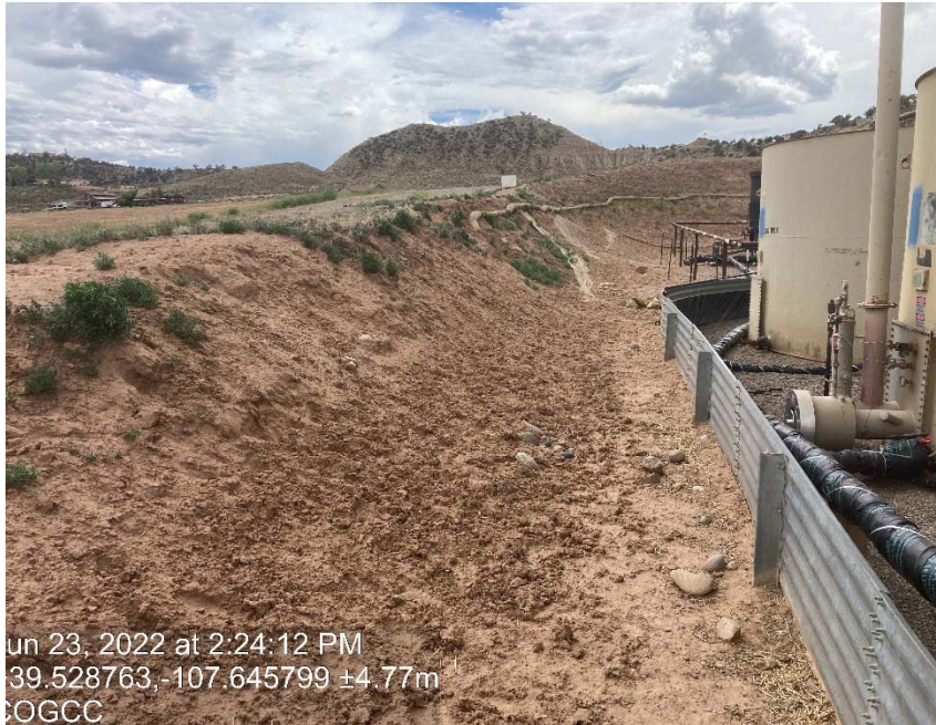
Lack of stabilization/ erosion/ debris
