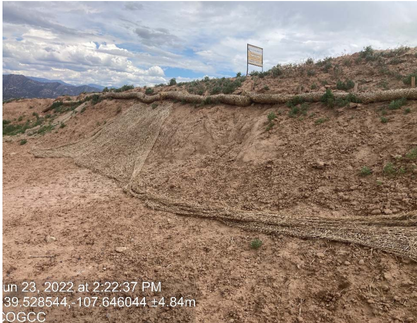
Lack of stabilization/ erosion/ debris
