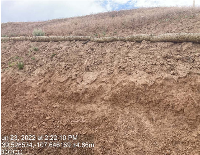
Lack of stabilization/ erosion
