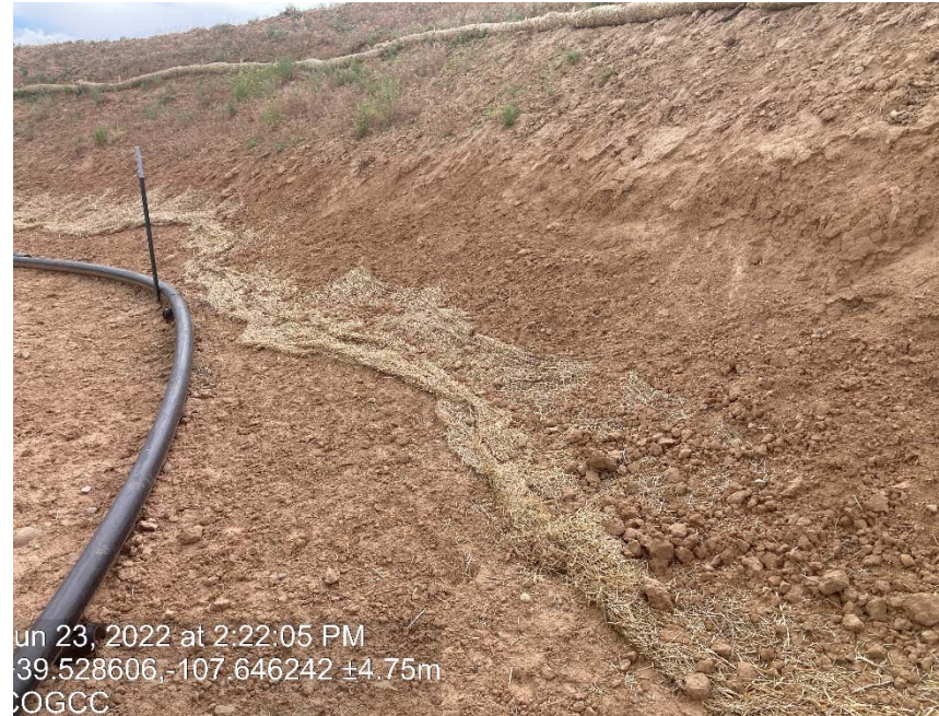
Lack of stabilization/ erosion/ debris
