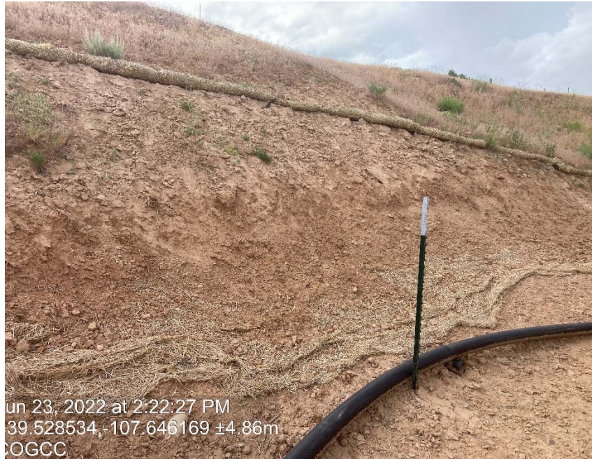
Lack of stabilization/ erosion/ debris
