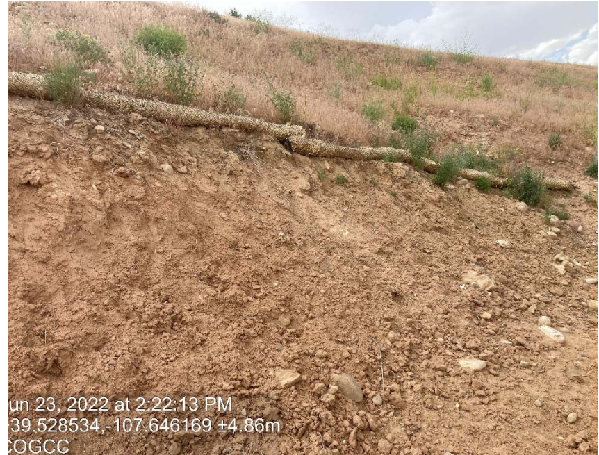
Lack of stabilization/ erosion
