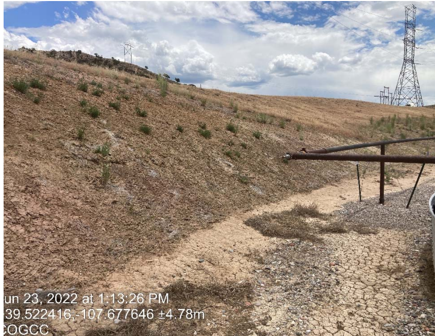
Lack of stabilization/ erosion
