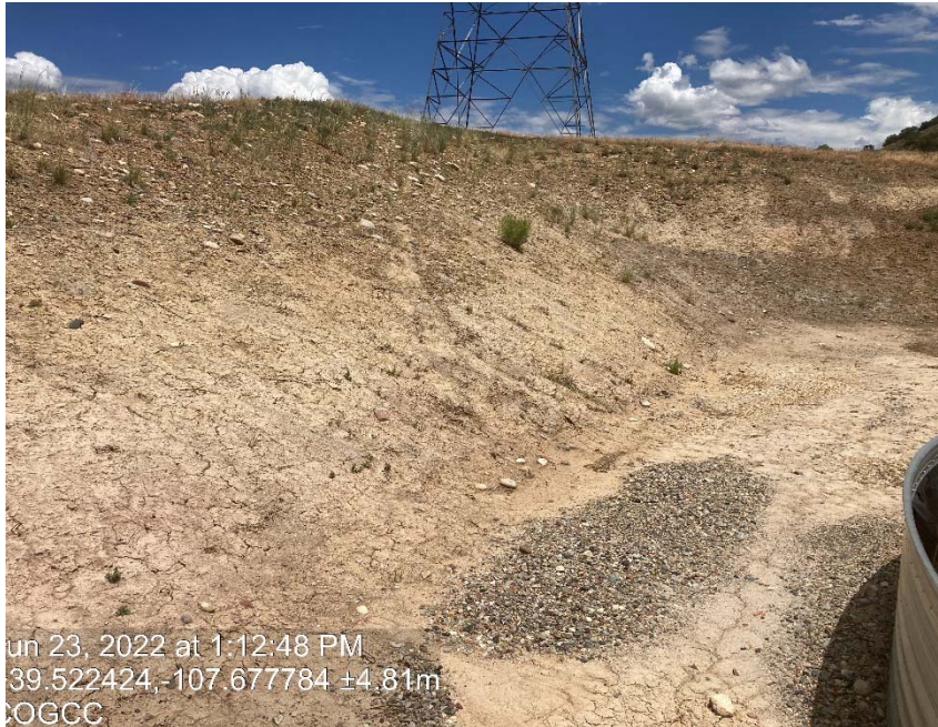
Lack of stabilization/ erosion
