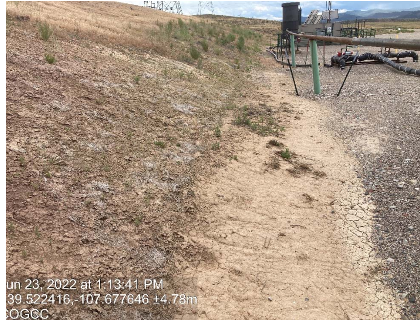
Lack of stabilization/ erosion
