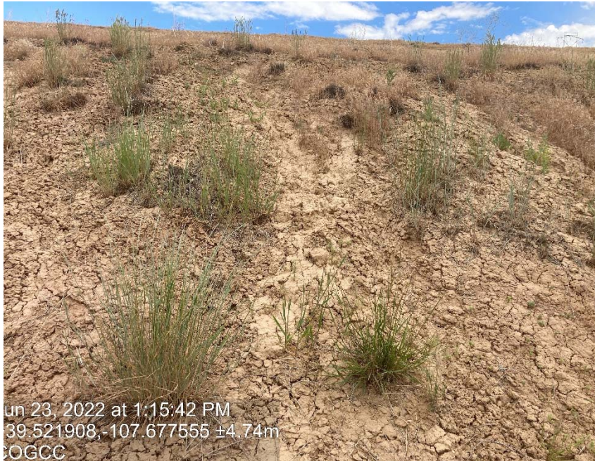
Lack of stabilization/ erosion
