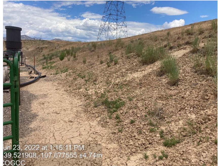
Lack of stabilization/ erosion
