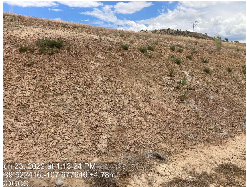
Lack of stabilization/ erosion
