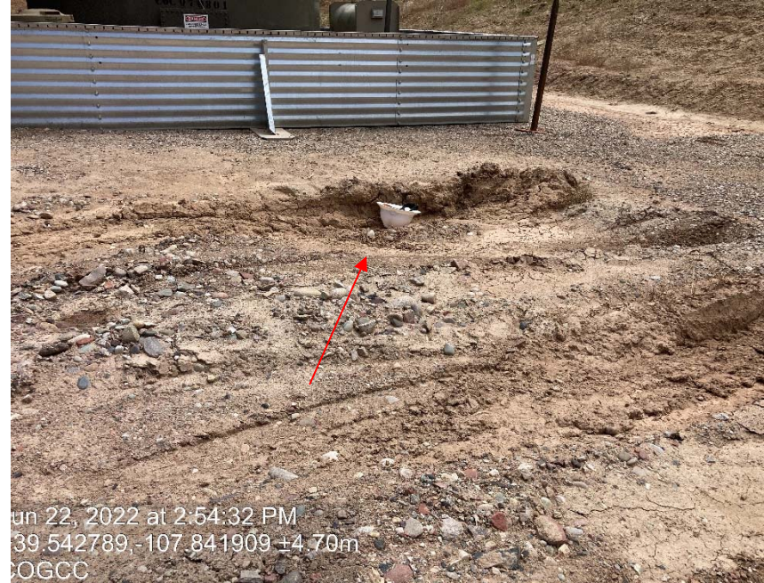
Lack of stabilization/compaction. Hard hat in photo for reference.
