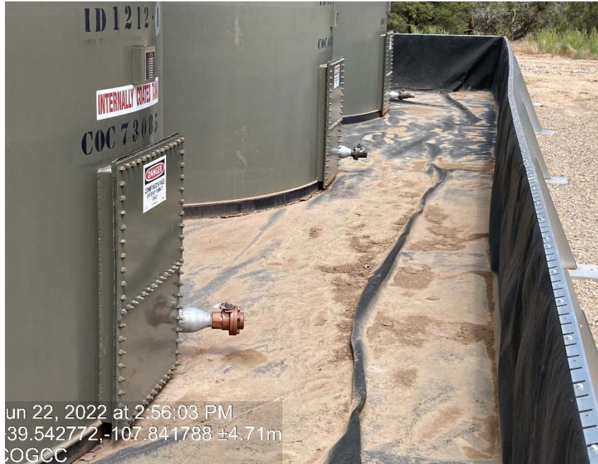
Two tanks are missing cap/plugs and third tank has plug/cap in photo
