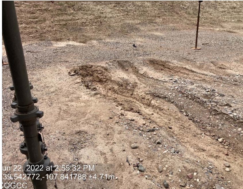
Lack of stabilization/compaction
