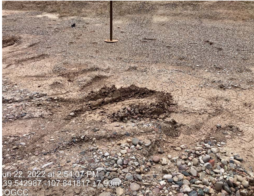
Lack of stabilization/compaction
