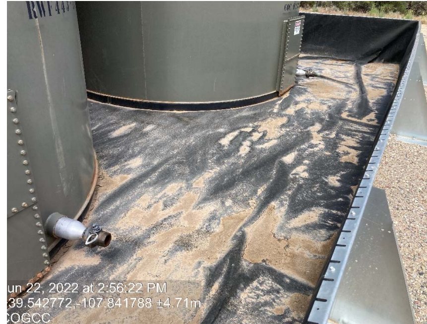
One tank is missing cap/plug and second tank has plug/cap in photo
