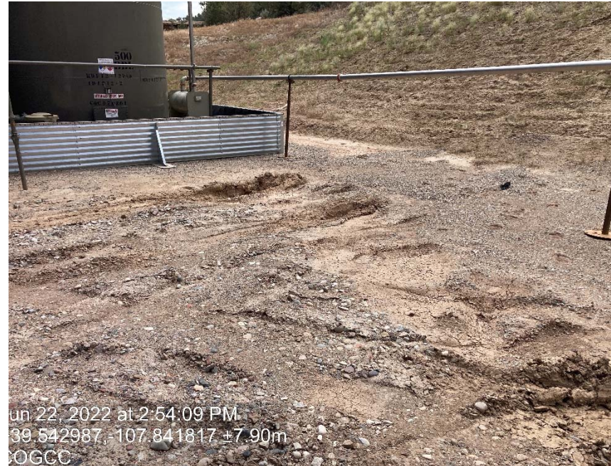
Lack of stabilization/compaction
