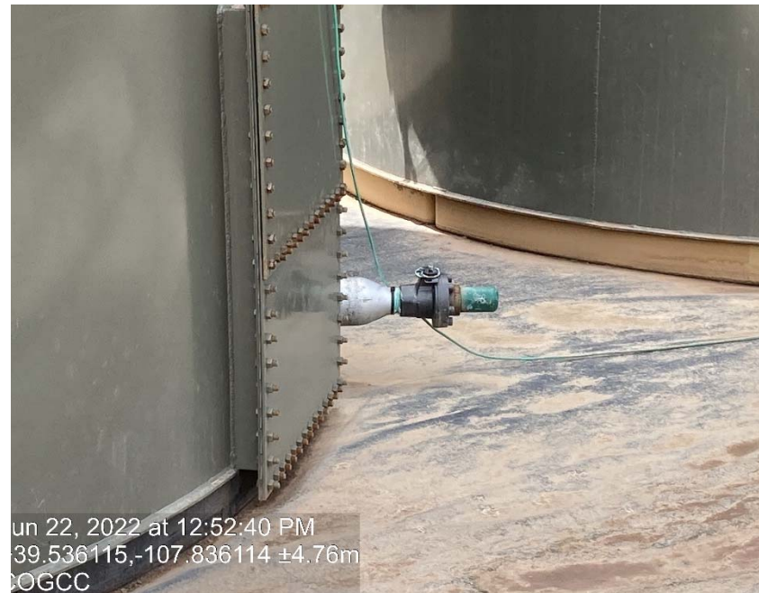
Valve on tank with plug/cap
