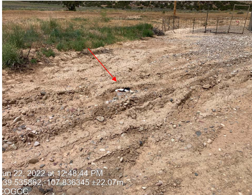
Lack of stabilization/ compaction. Hard hat in photo
