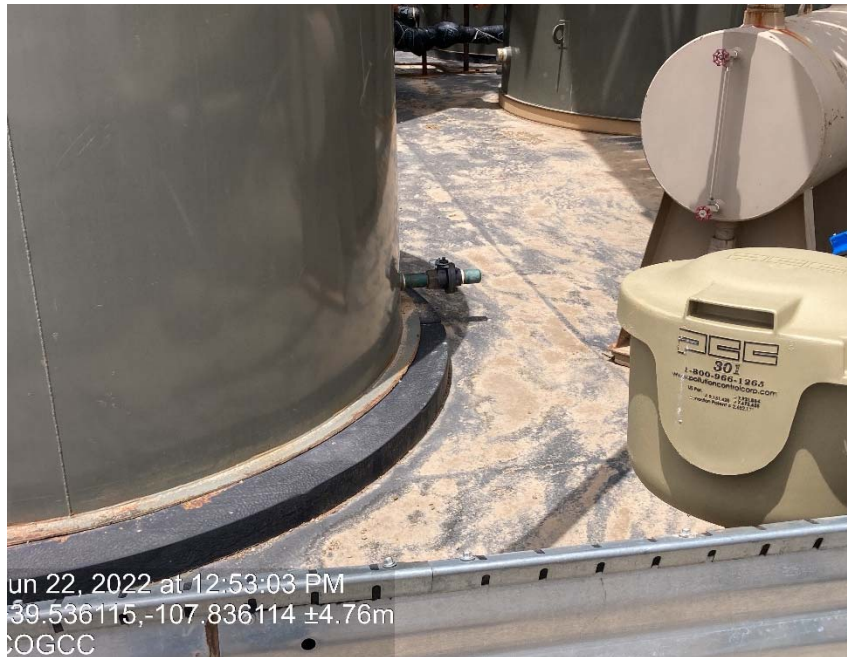
Valve on tank with plug/cap
