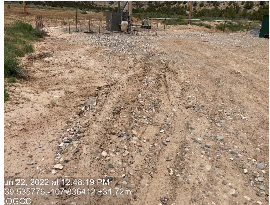
Lack of stabilization/ compaction
