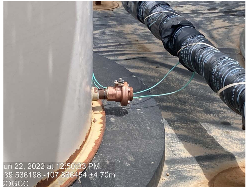
Valve on tank missing cap/plug
