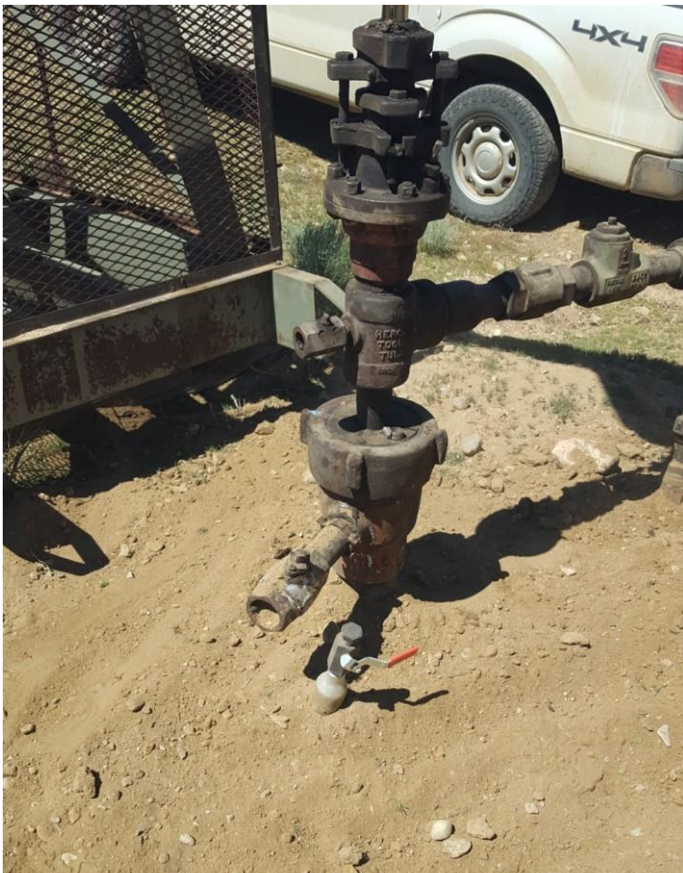
Figure #1 Bradenhead access has been installed.
