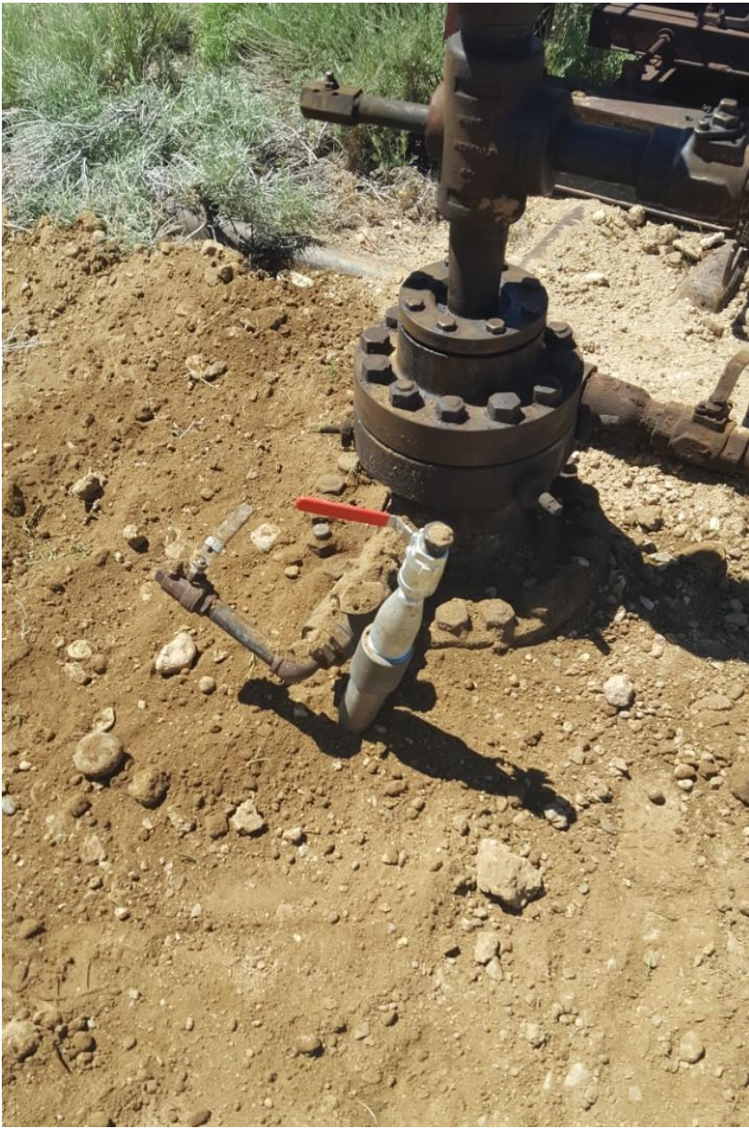
Figure #1 Bradenhead access has been installed.
