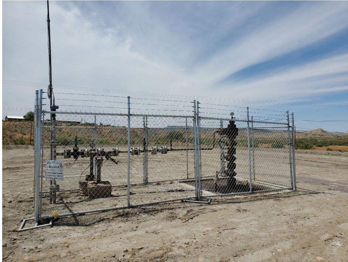
Injection wellhead.
