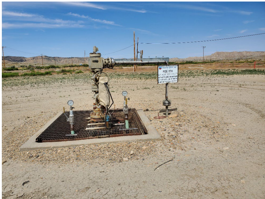
Injection wellhead.
