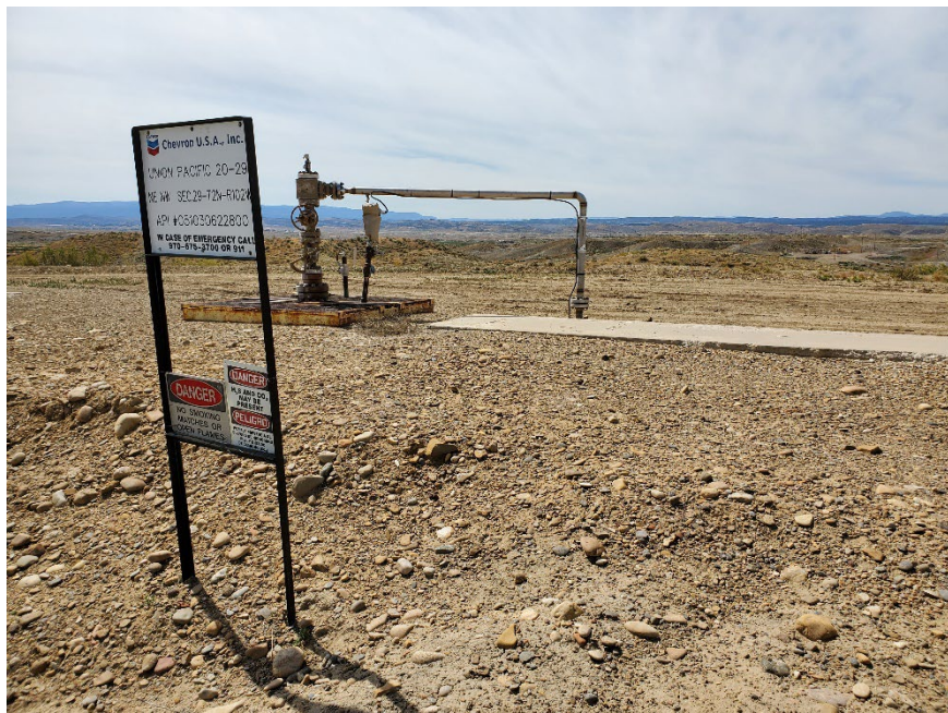
Injection wellhead
