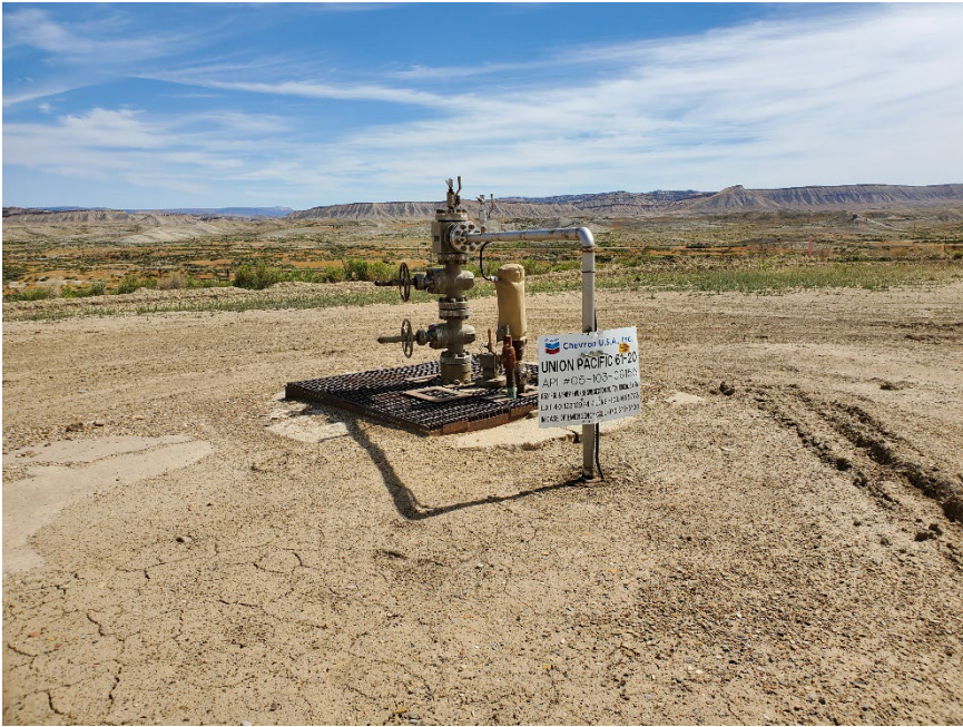
Injection wellhead
