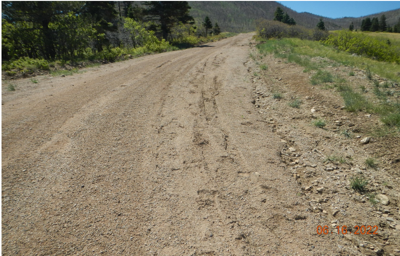
Photo 1. Facing south along the access road. There are some signs of erosion along the steep grade of the road. Stormwater should be diverted off the road to reduce erosion.
