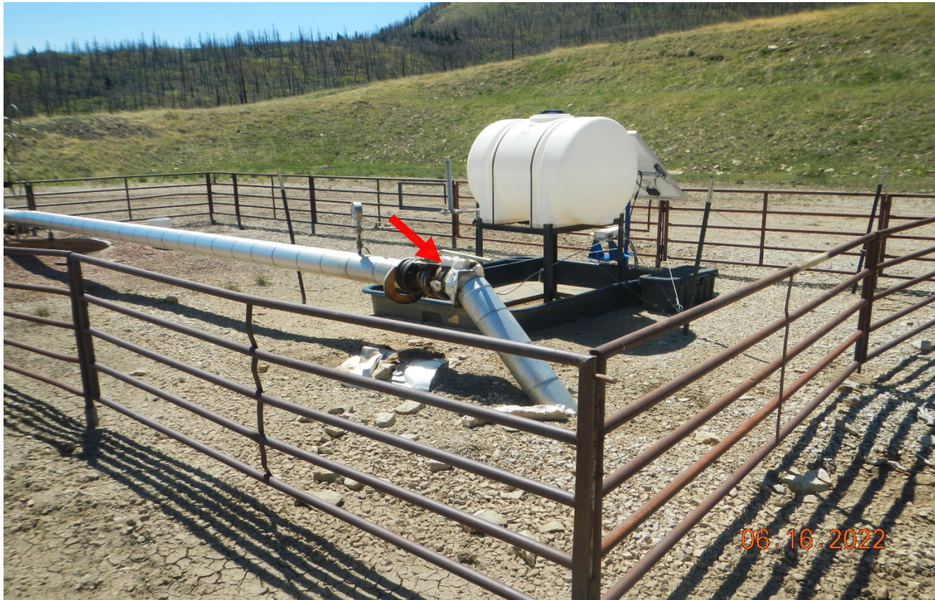
Photo 4. There was an audible gas leak. Gas monitor also detected a leak. Operator was notified by phone call of this issues.
