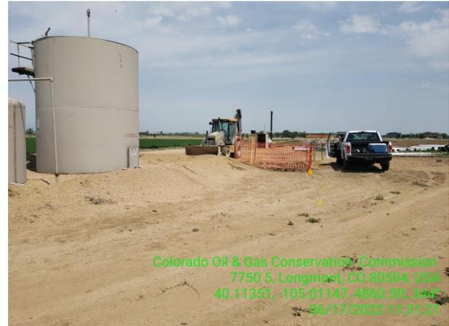
**Photo 9 Damaged flow line excavation.**
