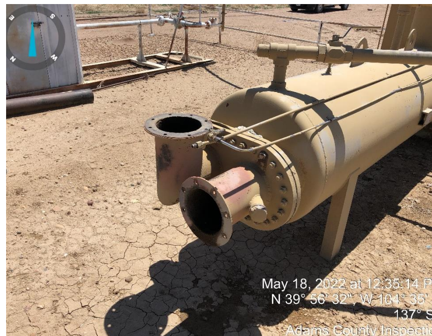
Photo #6 No wildlife protection on open equipment.
