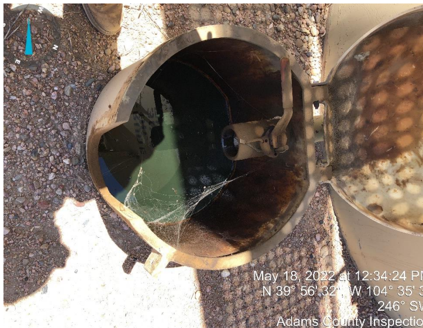
Photo #3 loadout line missing bull plug.
