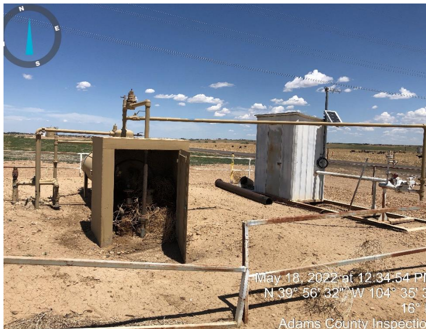
Photo #5 Separator and meter house.
