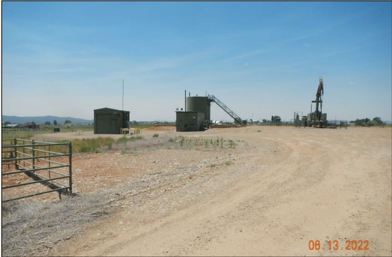
Photo 1. View of the project are from the well pad entrance facing center.
