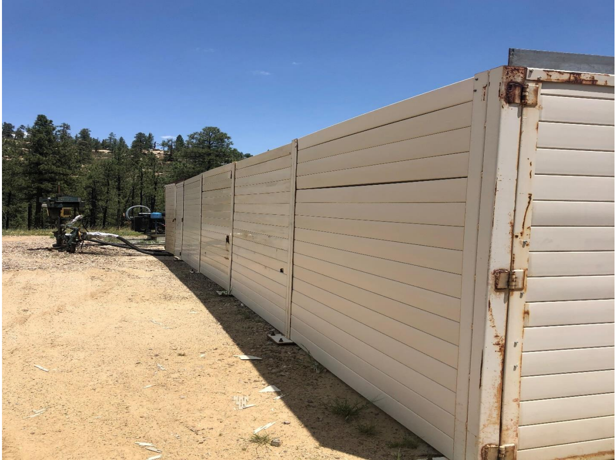
Repaired sound wall panels to comply with Rule 606
