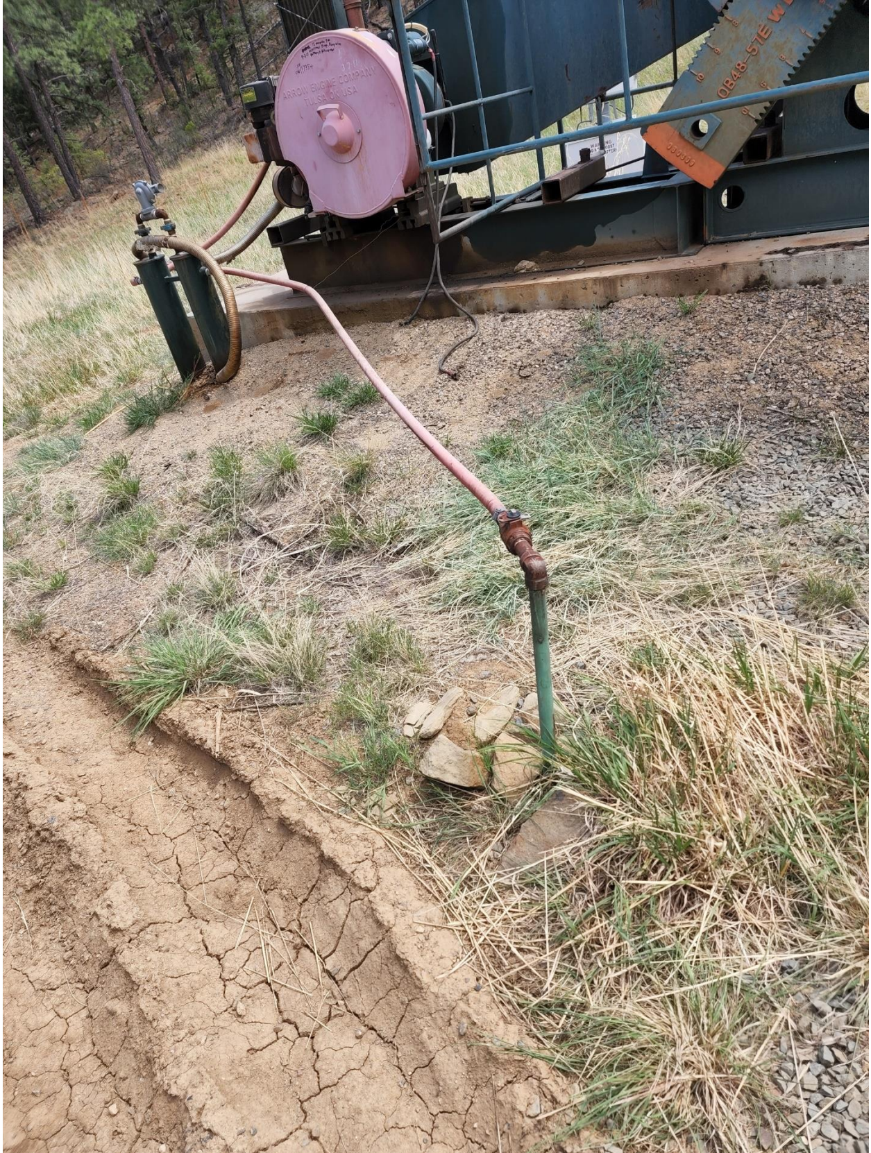
Repaired and put riser unuse per Rule 606.
