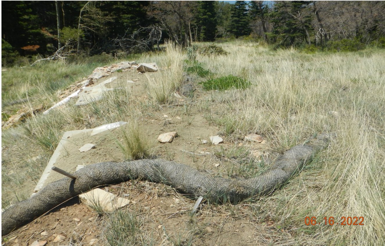
Photo 3. There are some displaced straw wattles at the spring area at the northwest side of the location.
