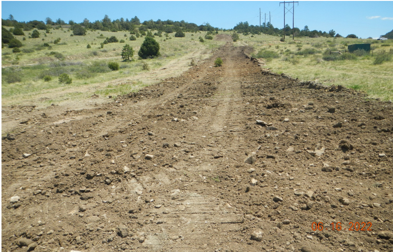
Photo 5. Facing east toward the flowline disturbance between the meter station and compressor. All soils will need to be replaced, reclaimed, and stabilized.
