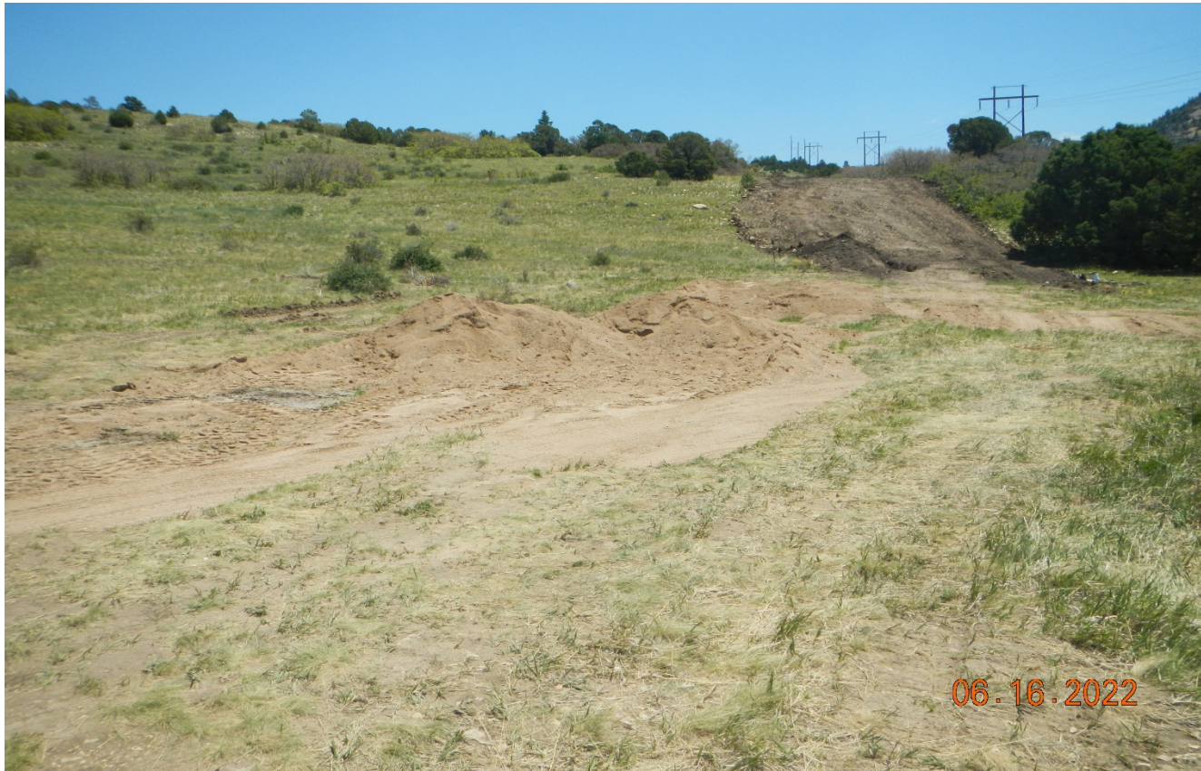
Photo 1. Facing southeast. There has been disturbance along the flowline from the Compressor to the meter station. There is a pile of sand fill material that will need to be removed. All soils will need to be replaced, reclaimed, and stabilized.
