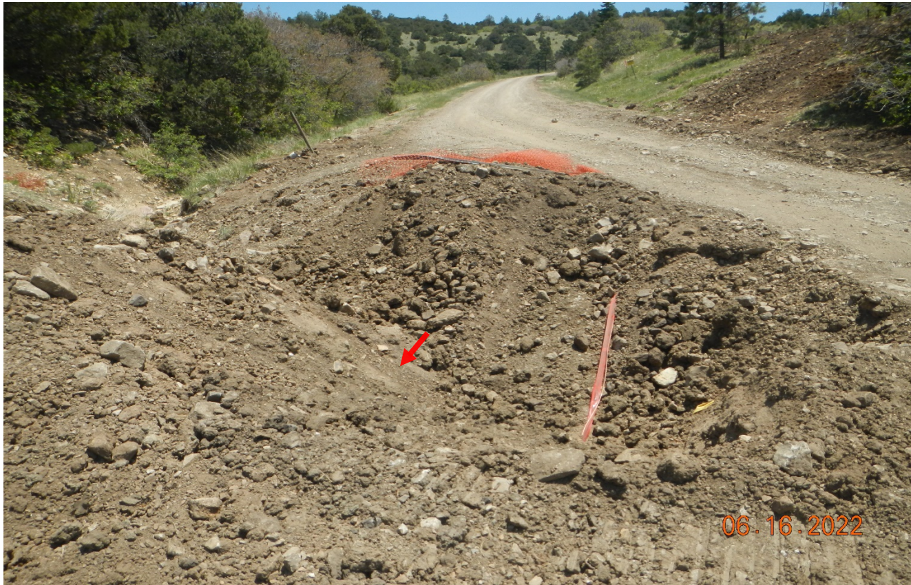
Photo 3. The flowline crossed the road at this point. The orange safety fence is not maintained and there is a large excavated I the road way.
