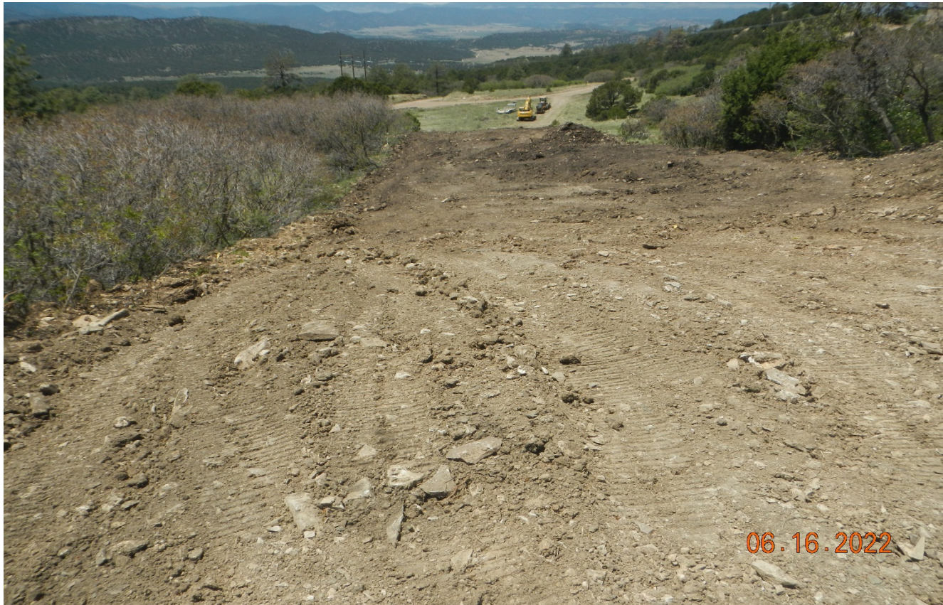
Photo 2. Facing back to the northwest along the flowline disturbance. All soils will need to be replaced, reclaimed, and stabilized.
