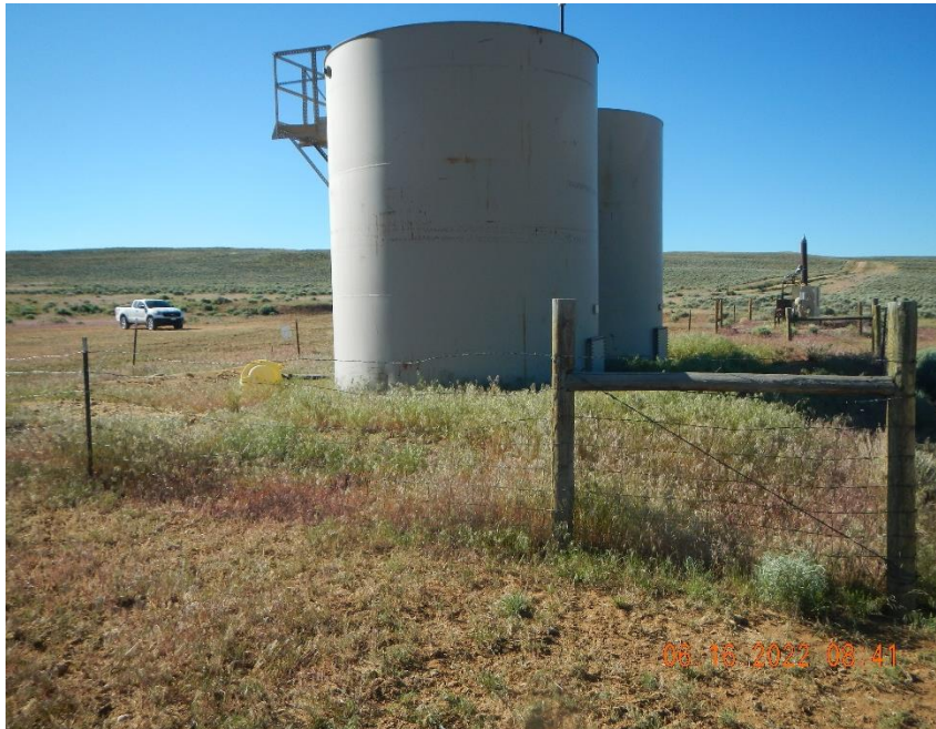
Weeds growing inside of tank battery berm.
