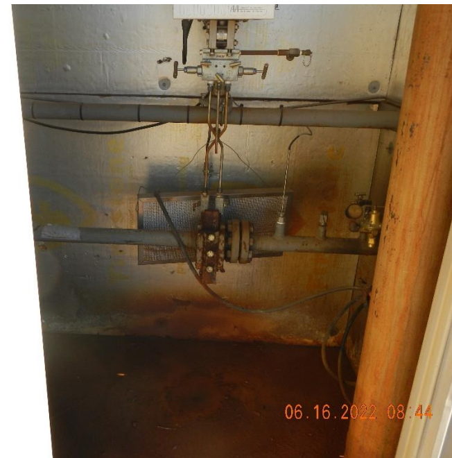
Leak at orifice plate inside of meter shed.
