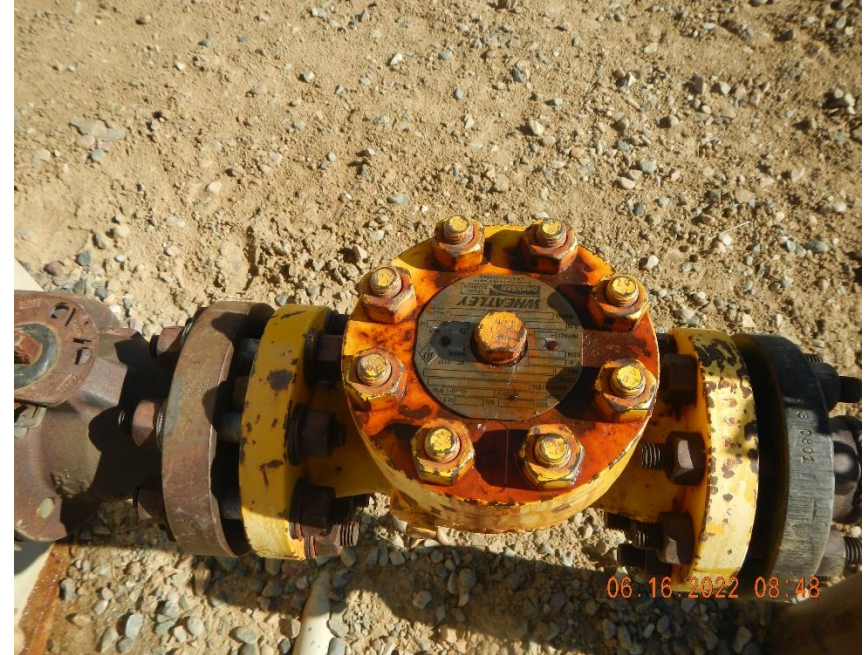
Yellow 2" valve outside of metershed is wet from leak around stem.
