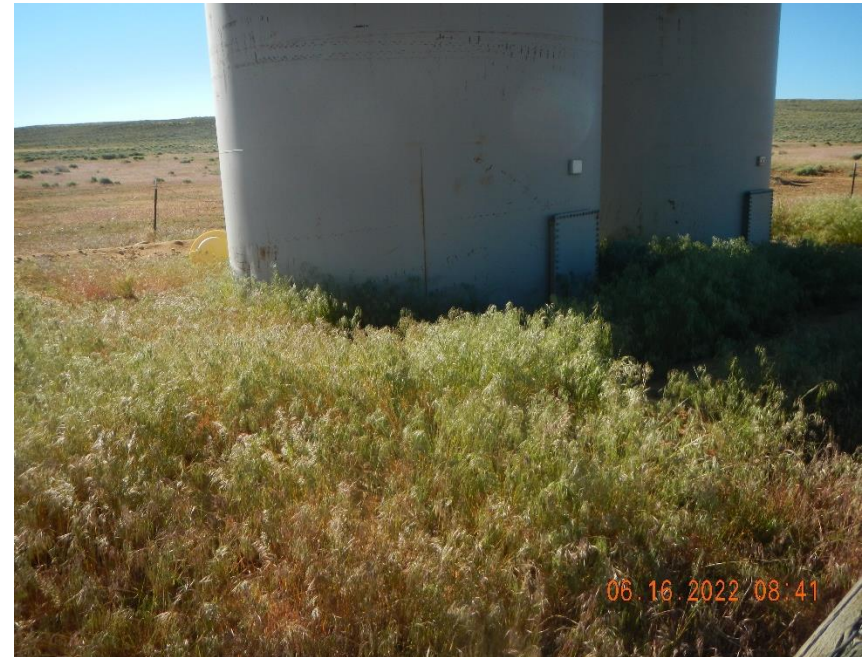
Weeds growing inside of tank battery berm.
