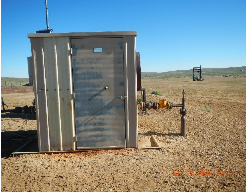
Yellow 2" valve outside of metershed is wet from leak around stem.
