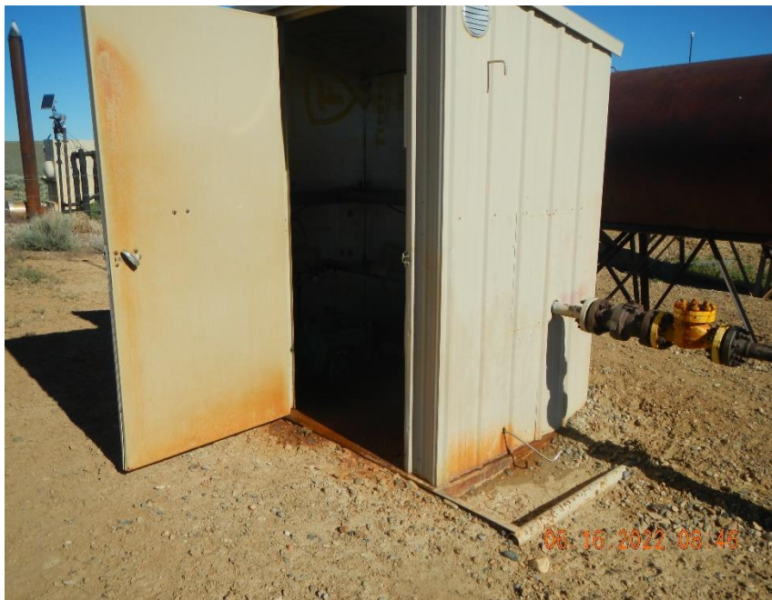
Leak at orifice plate inside of meter shed.
