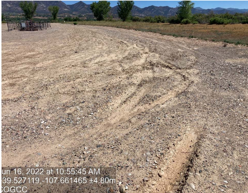
Lack of stabilization/ compaction
