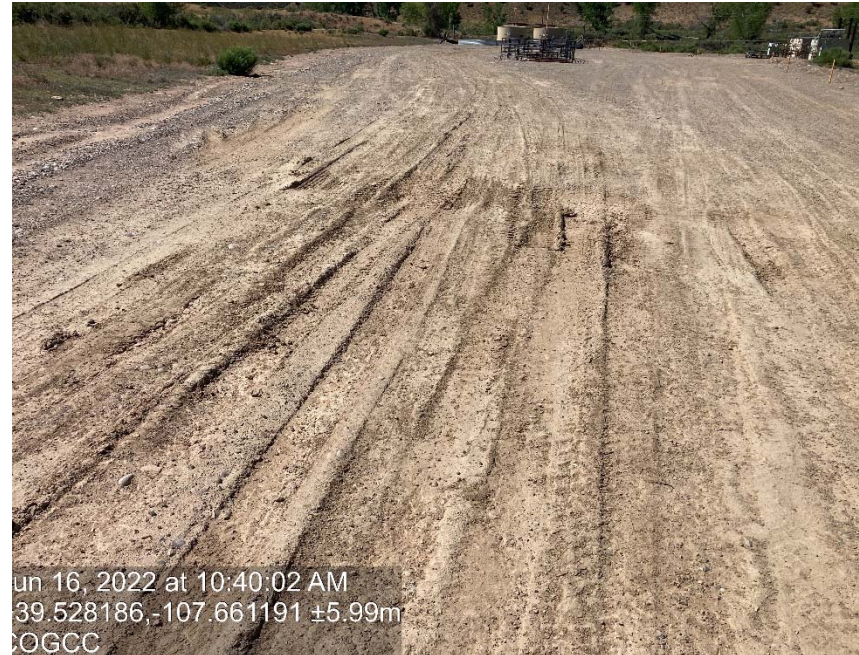
Lack of stabilization/ compaction
