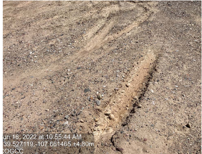
Lack of stabilization/ compaction
