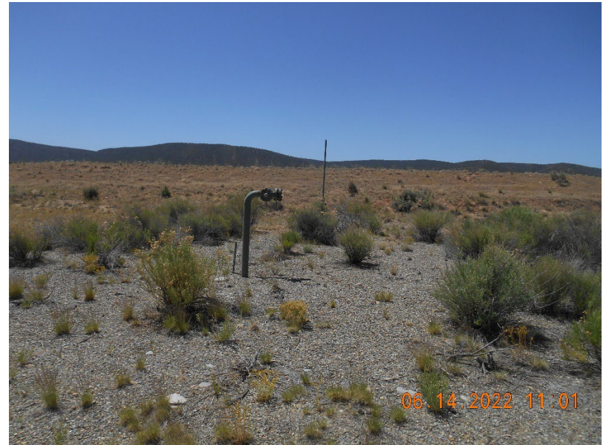
Flowline riser locked out/tagged out Unused flowlines removed
