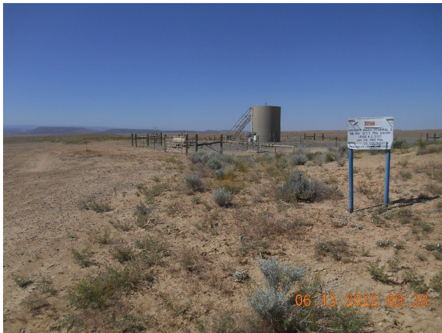
Location overview looking S.
