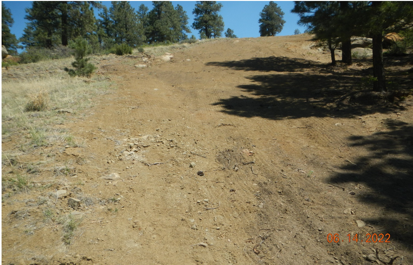
Photo 1. Facing northeast at the disturbance along the gathering pipeline at Lat/Long:37.05440,-104.76614. This area has been reseed however, soils are not stabilized and are susceptible to erosion.
