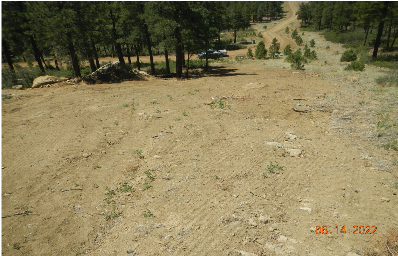
Photo 2. Facing southwest along the pipeline disturbance. The disturbed soils are susceptible to erosion due to seep conditions and lack of stabilization until vegetation establishes.
