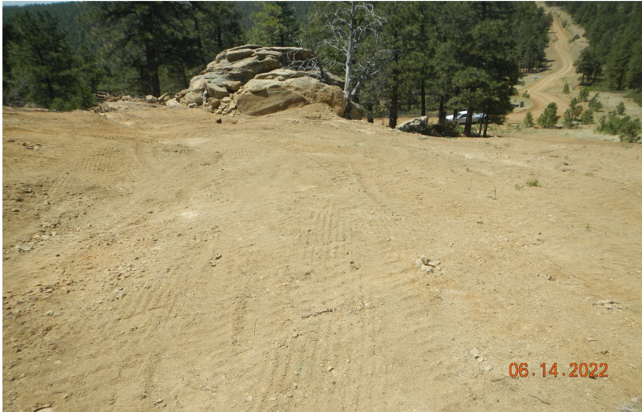
Photo 3. Facing southwest along the pipeline disturbance. The disturbed soils are susceptible to erosion due to seep conditions and lack of stabilization until vegetation establishes.
