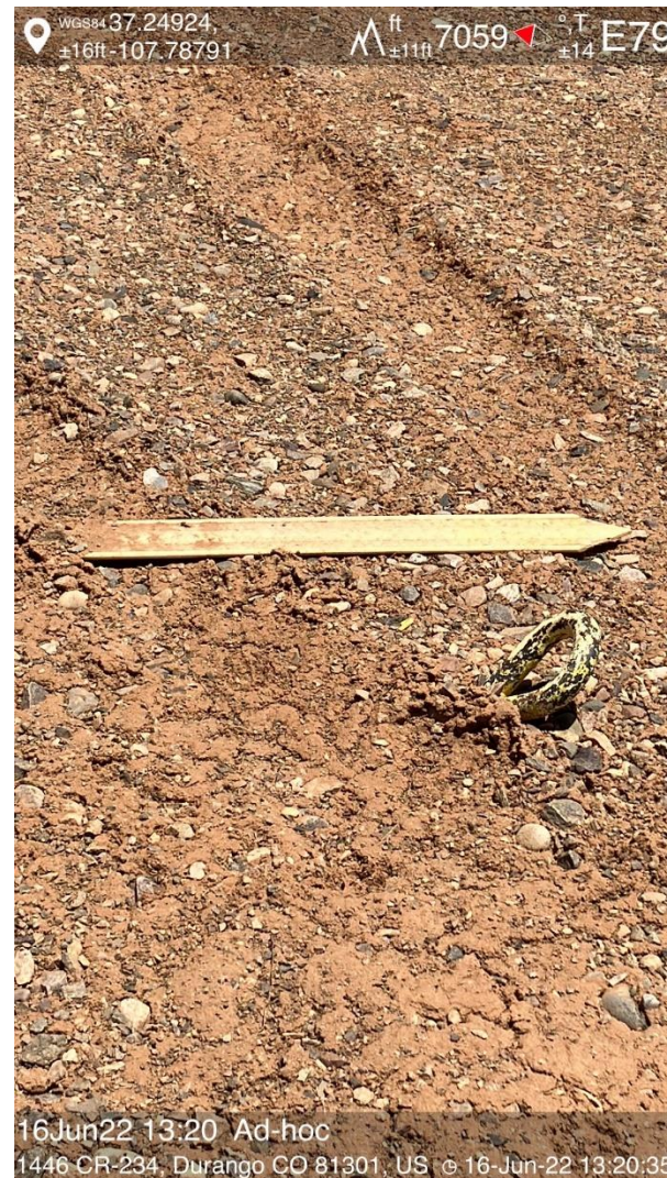
IMG 06 Rig anchor not secured
