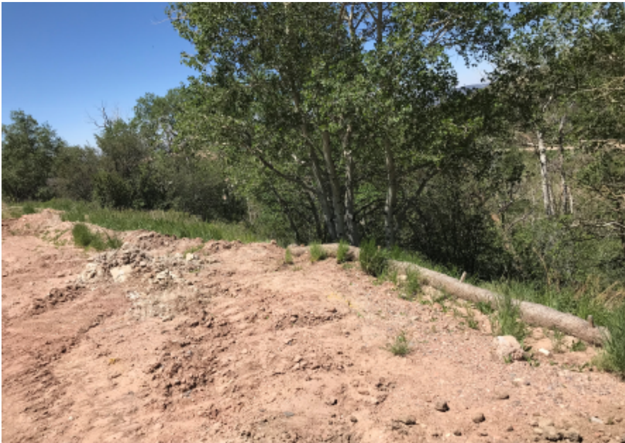
Waddles have been repaired or replaced to control sediment.
