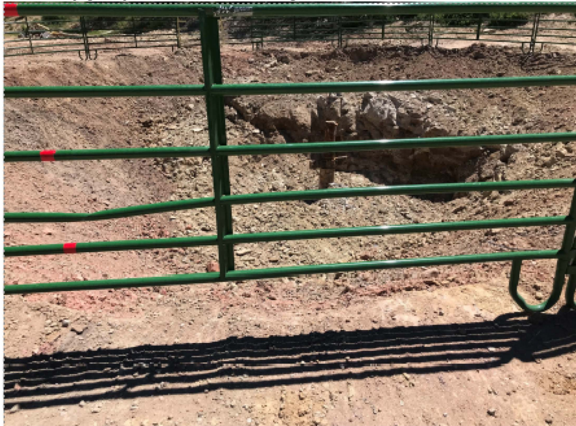
Photo taken from the center of the Location shows the excavation around the wellhead. Fence panels completely enclose the area and the slope of the pit is sufficiently gently to allow for wildlife egress
