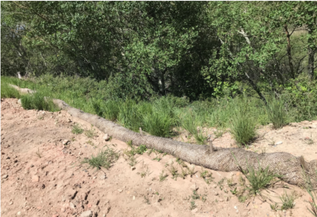
Waddles have been repaired or replaced to control sediment.
