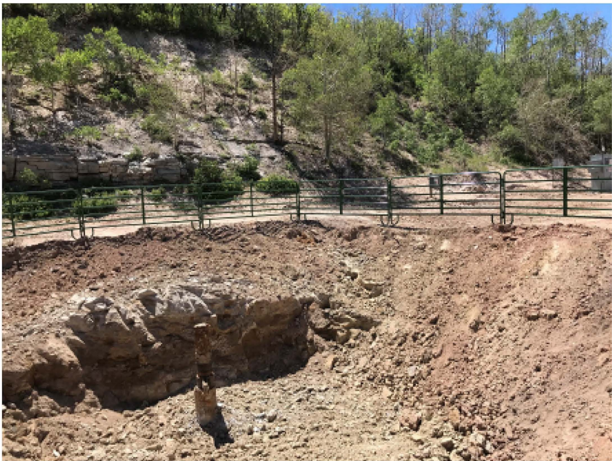
Photo taken from the center of the Location shows the excavation around the wellhead. Fence panels completely enclose the area and the slope of the pit is sufficiently gently to allow for wildlife egress
