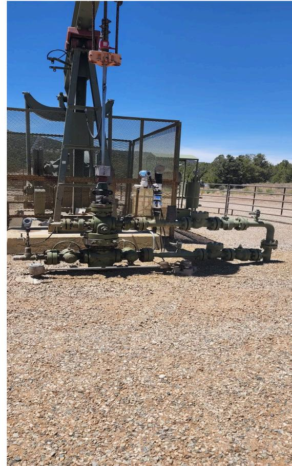
Remove stained soil from around separator piping
